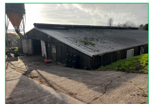
Developed land; sealed surface (agricultural building and adjacent hard standing)
