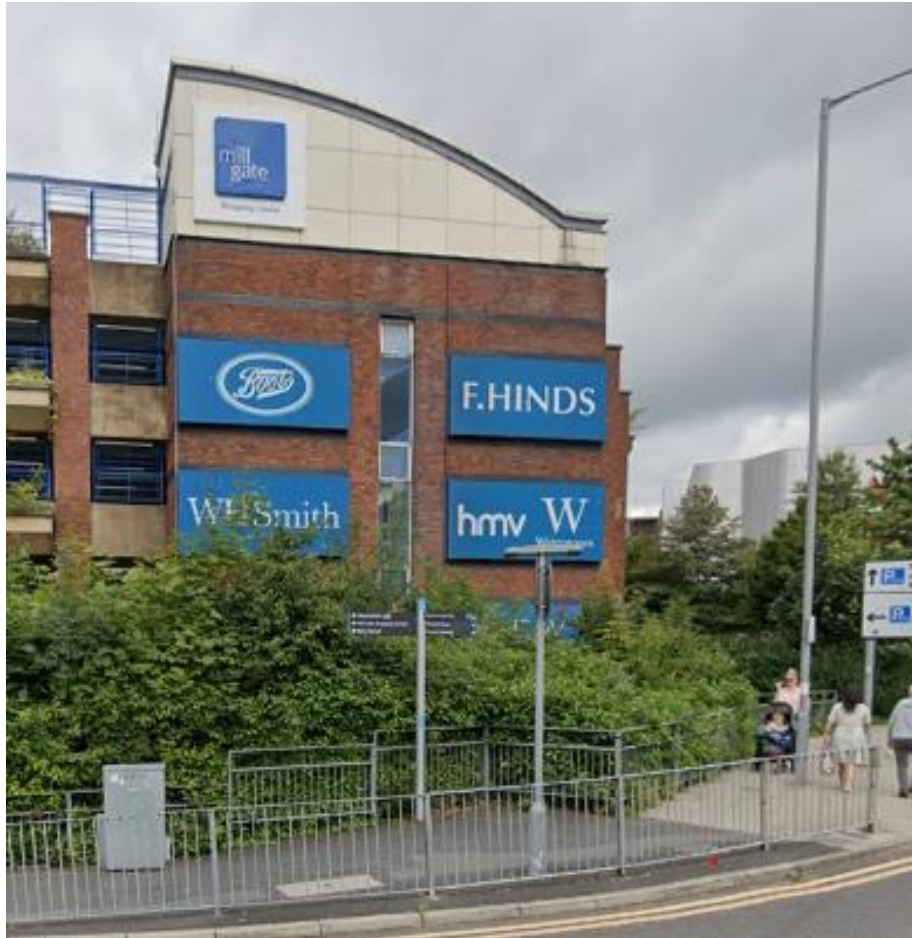
Prominent advertisement display at the multi-storey car park to the north
