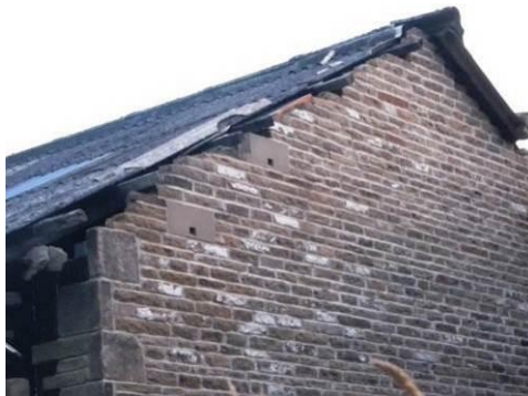
Example of Forticrete boxes in situ
