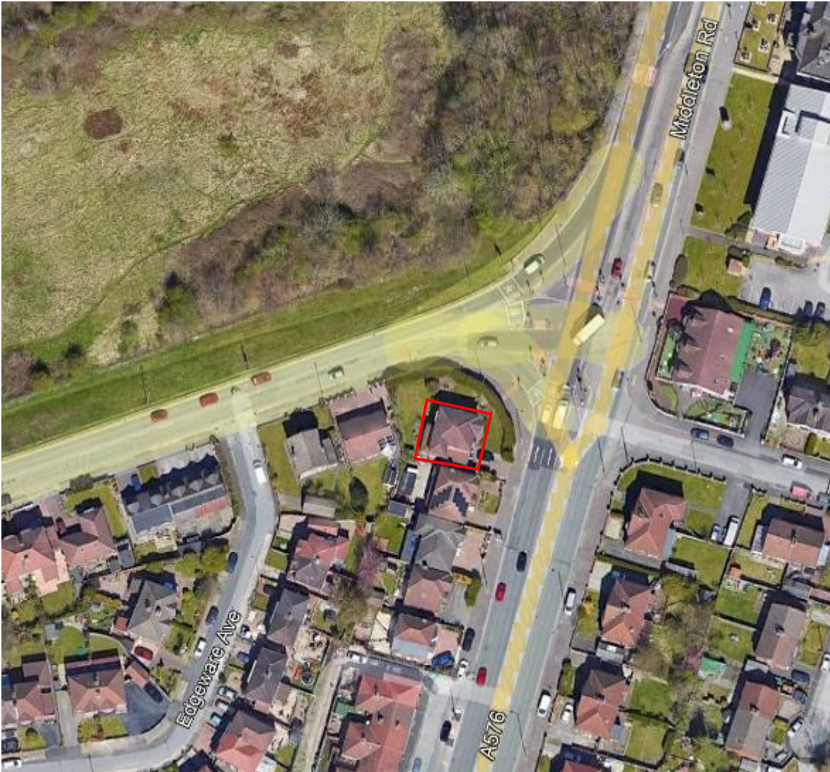
Figure 2: Aerial View of the Farmhouse Subject to Survey
