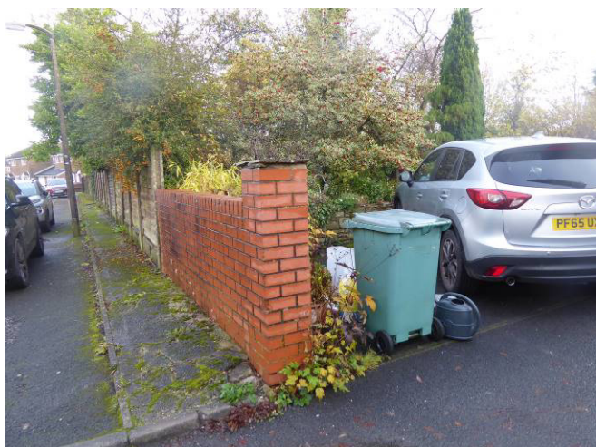
Southern entrance into the site and looking long the western boundary.
