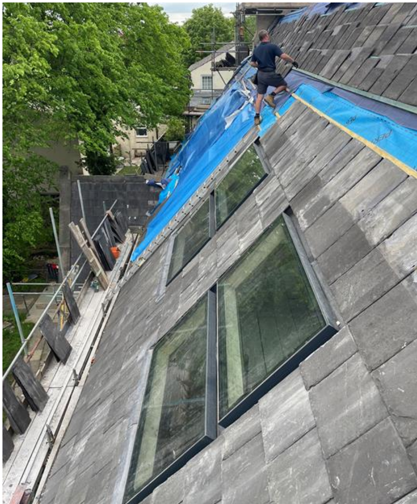
Figure 3.1: Applicant investment in repairing the roof.
