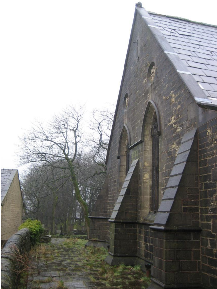
Figure 6.4: South Elevation prior to conversion.
