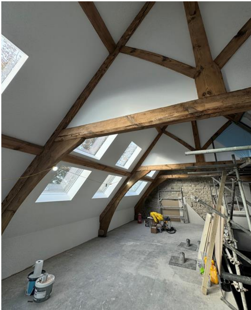
Figure 8.7: Investment in repair of historic timberwork
