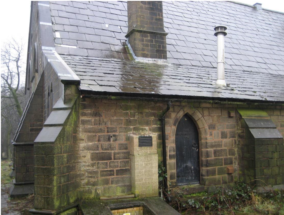
Plate 4: East elevation showing the porch doorway.
