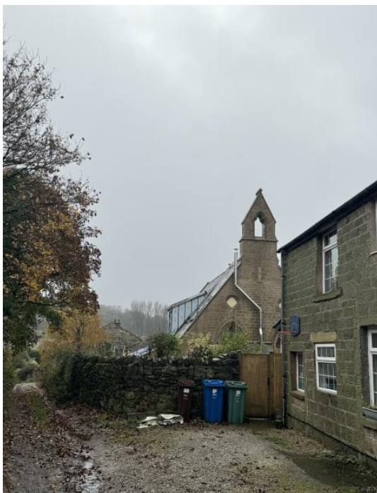
Figure 6.3: North Elevation, October 2024
