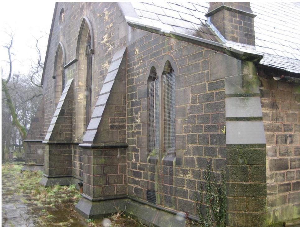
Plate 2: South elevation showing the aisle in the foreground.
