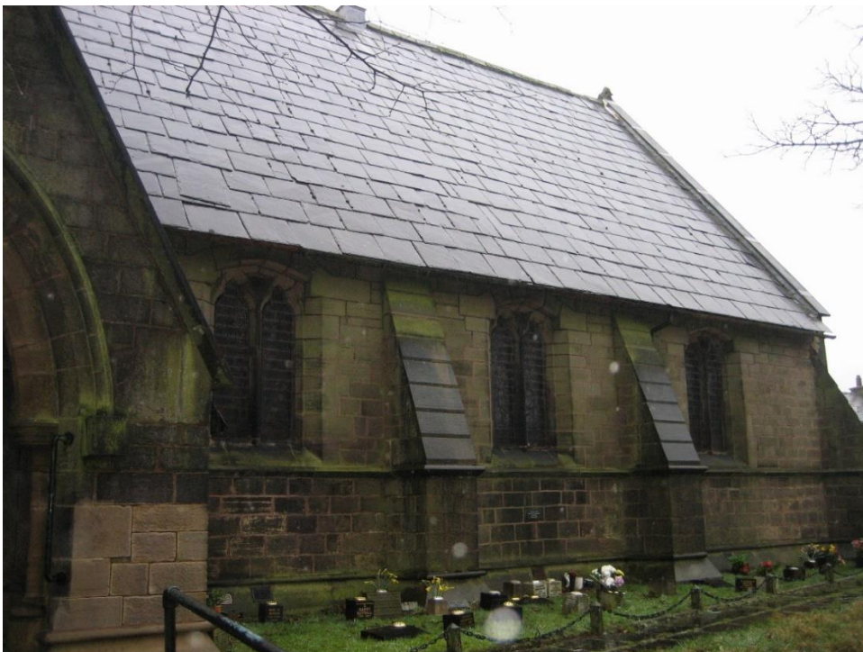
Plate 7: West elevation showing bays 3, 4 and 5.
