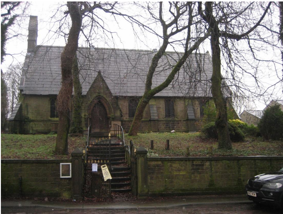
Plate 5: West elevation from Whalley Road.
