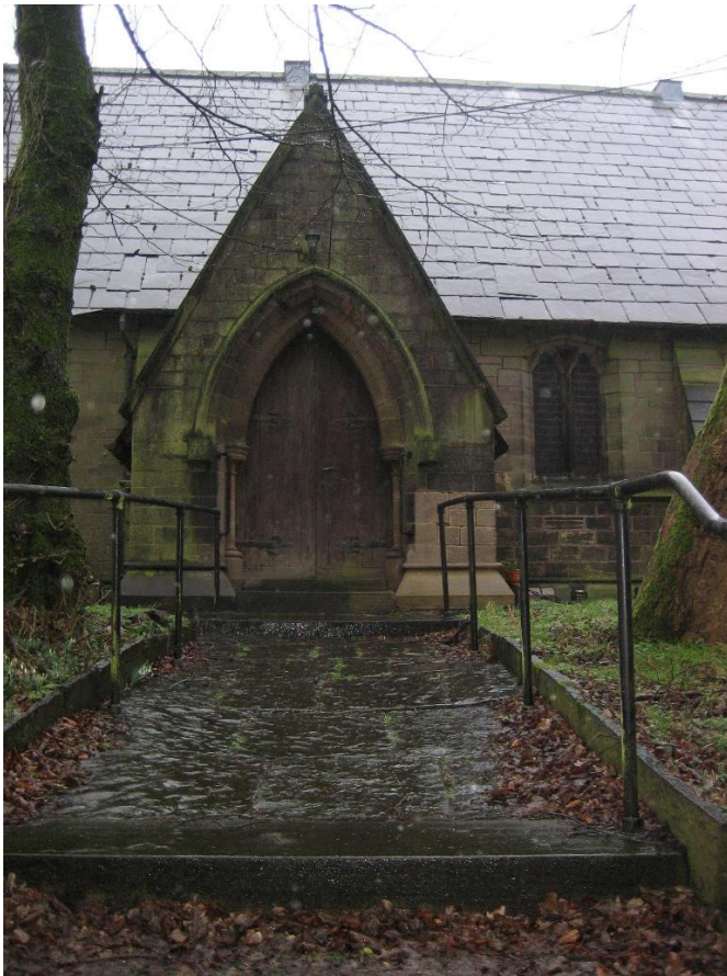
Plate 6: West elevation showing the porch at bay 2.
