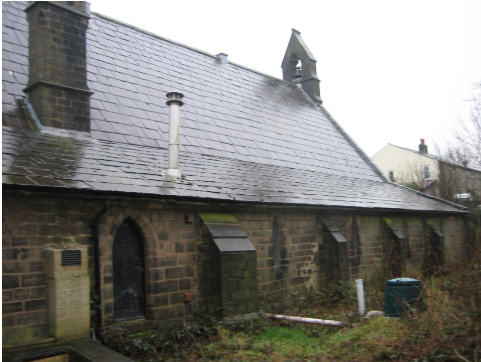
Figure 6.5: East Elevation prior to conversion.
