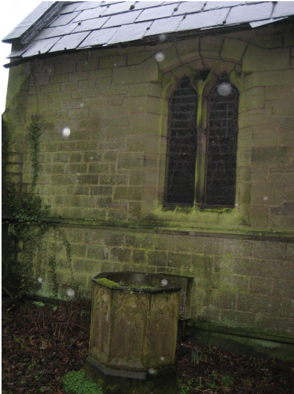
Plate 8: West elevation showing bay 1 with font in foreground.
