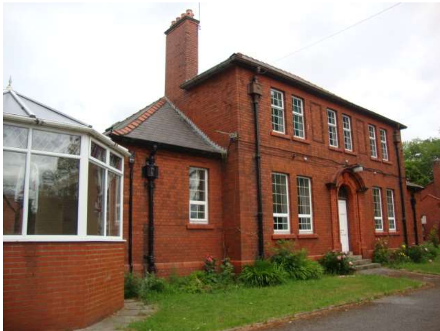
Figure 1 – Front elevation to Administration Block
