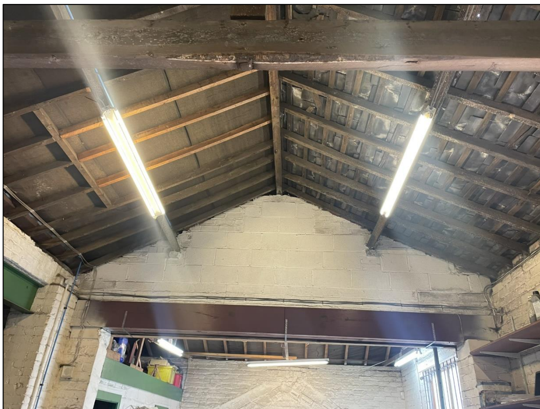
Plate 5 – General character of the roof, with partial Bitumen 1f lining beneath the roof and areas of no roof lining.
