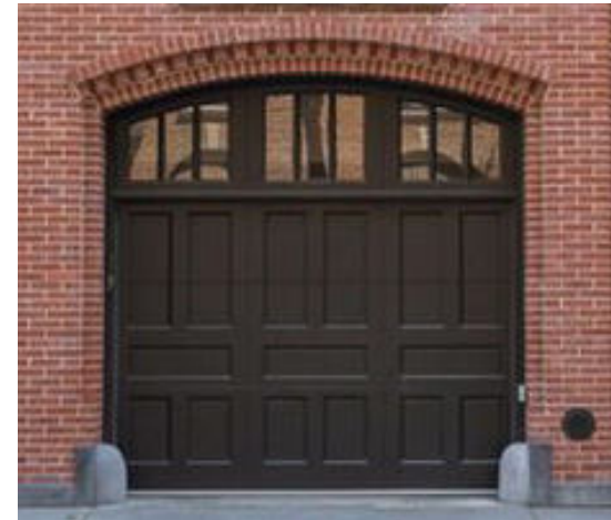
Timber doors to bin area with fanlight above
