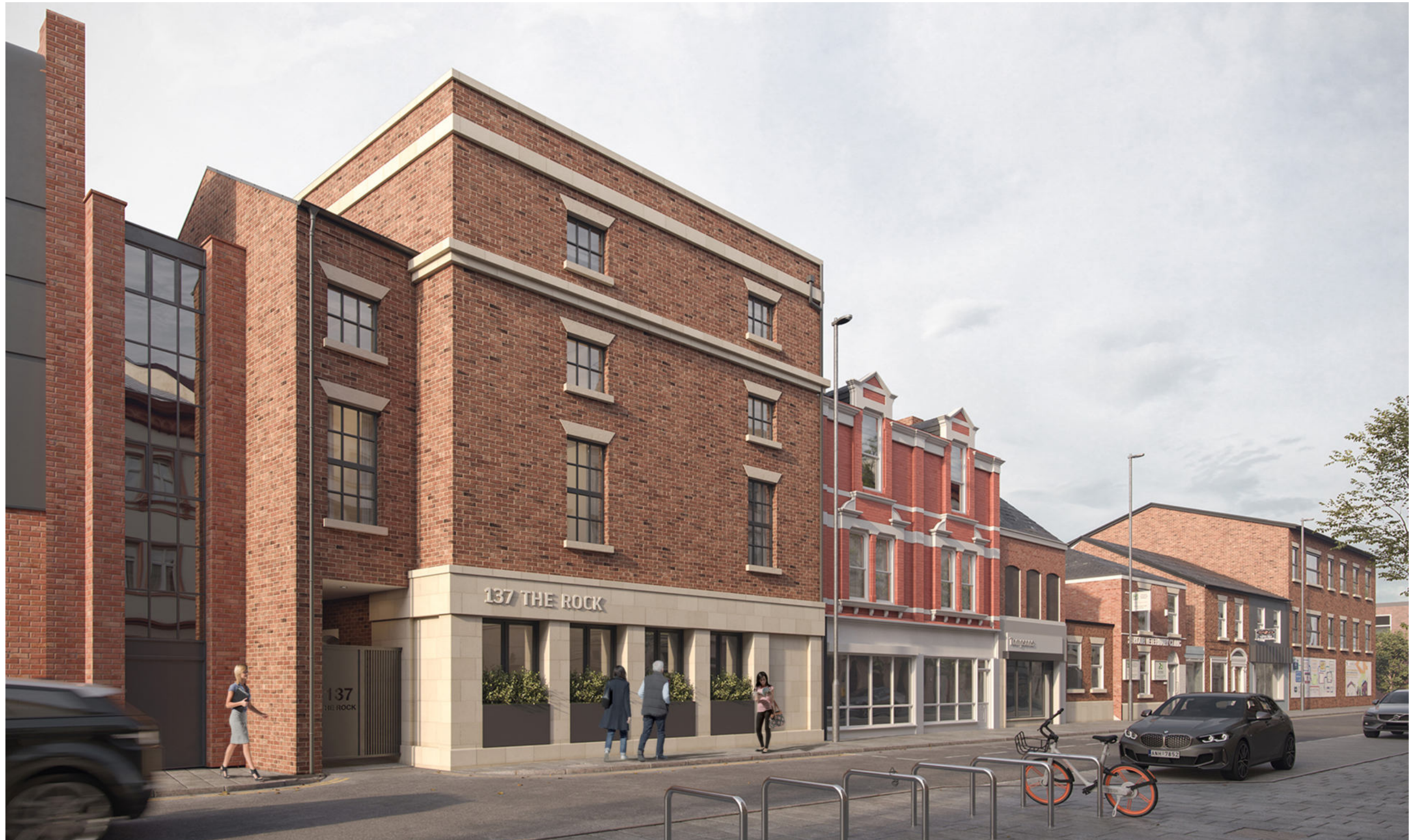
EXTERNAL VIEWS- FRONT STREET
