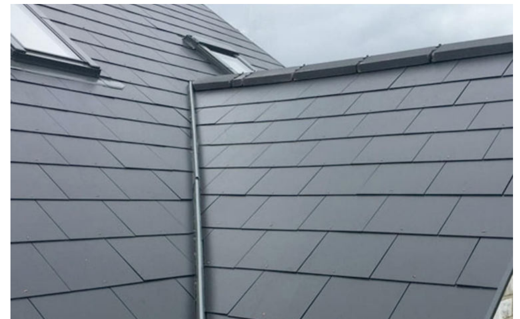
Fibre Cement Roof Tiles to houses
