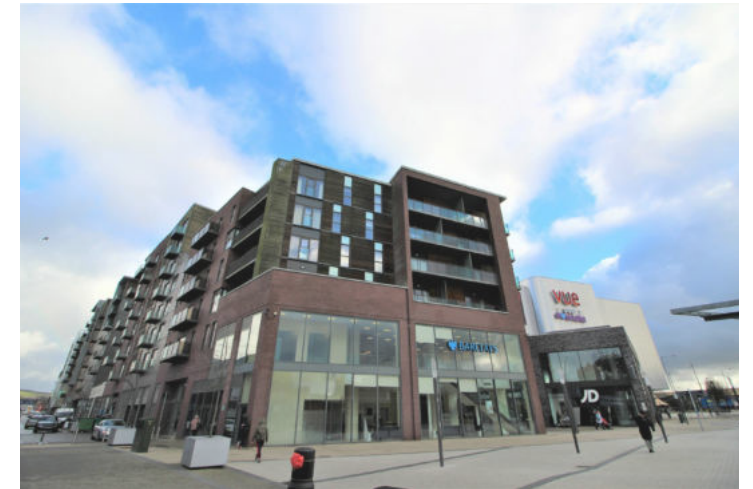
The Rock Accomodation
