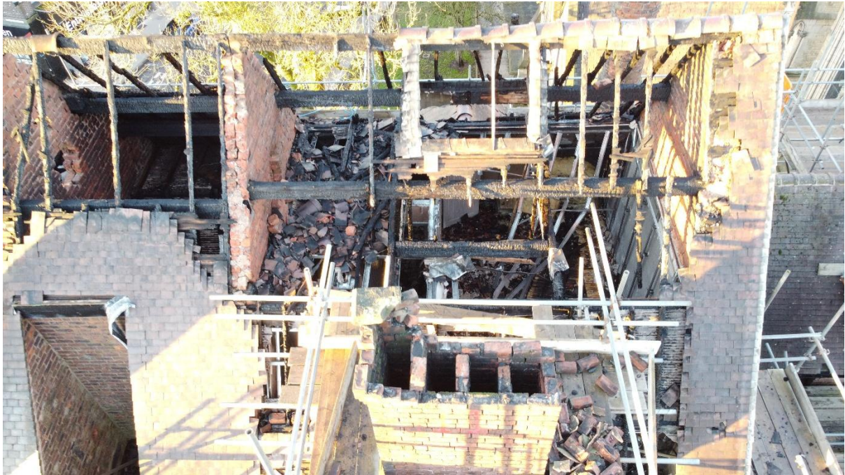
Picture 3 View On Roof - Rear Section
