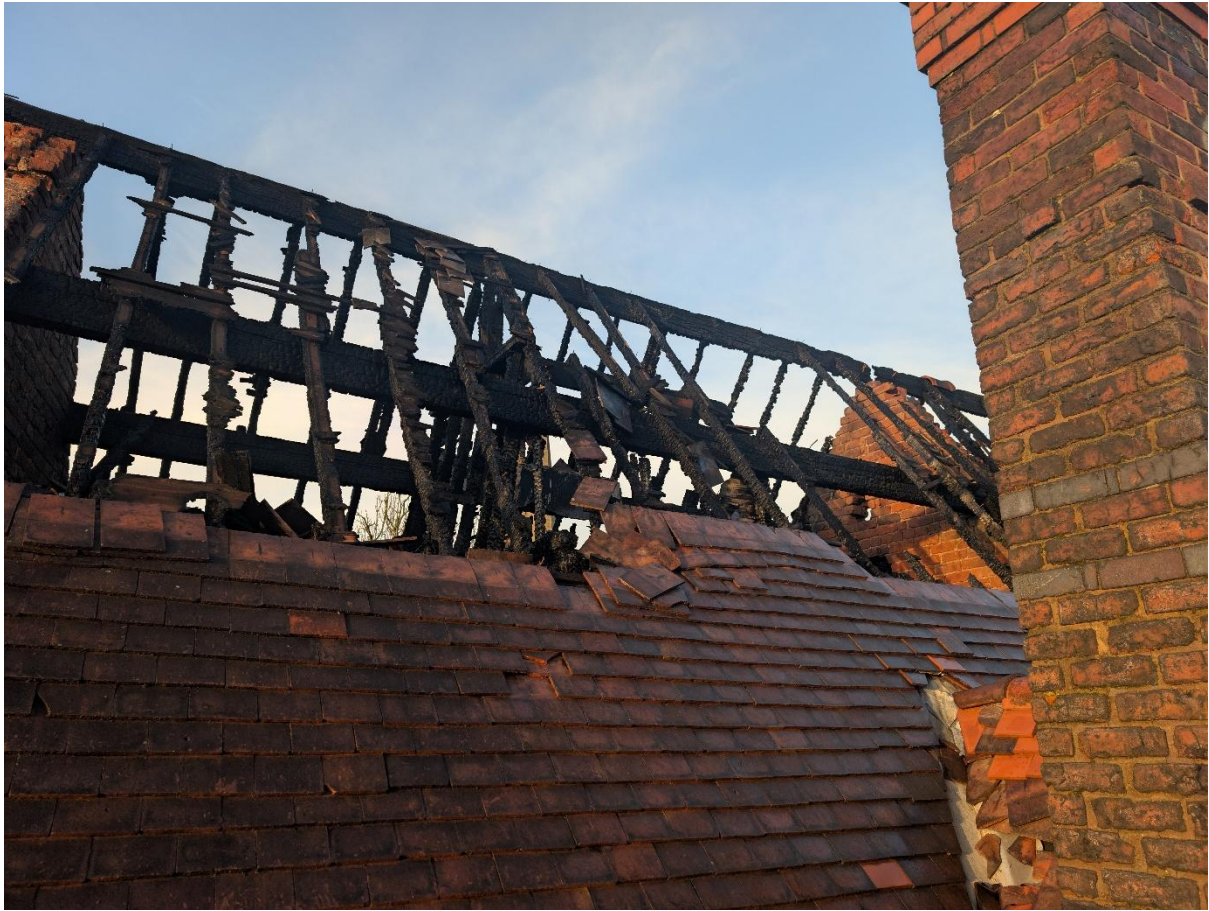
Picture 7 View On Roof
