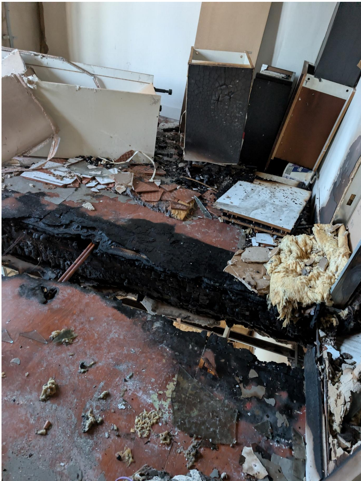
Picture 17 3rd Floor Rear Left Section
