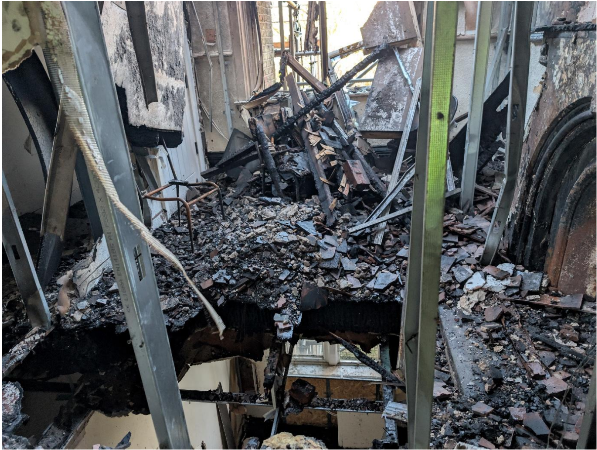
Picture 16 3rd Floor Rear Right - Possible Seat of Fire
