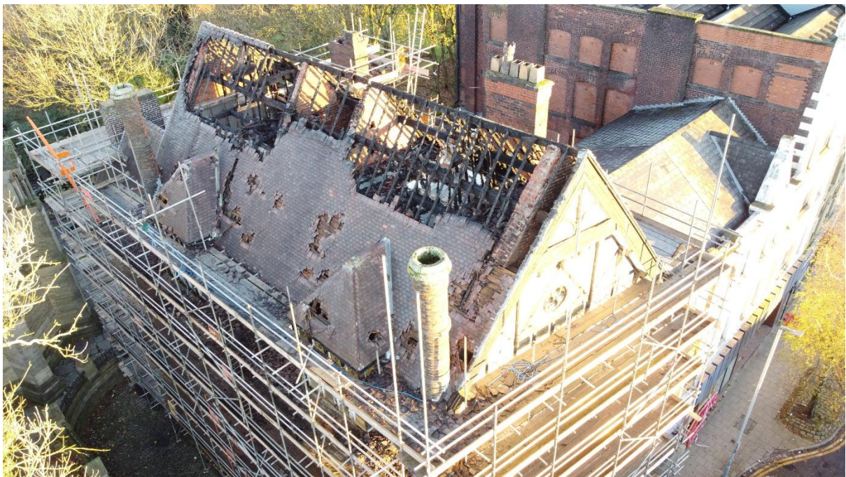
Picture 4 View On Roof
