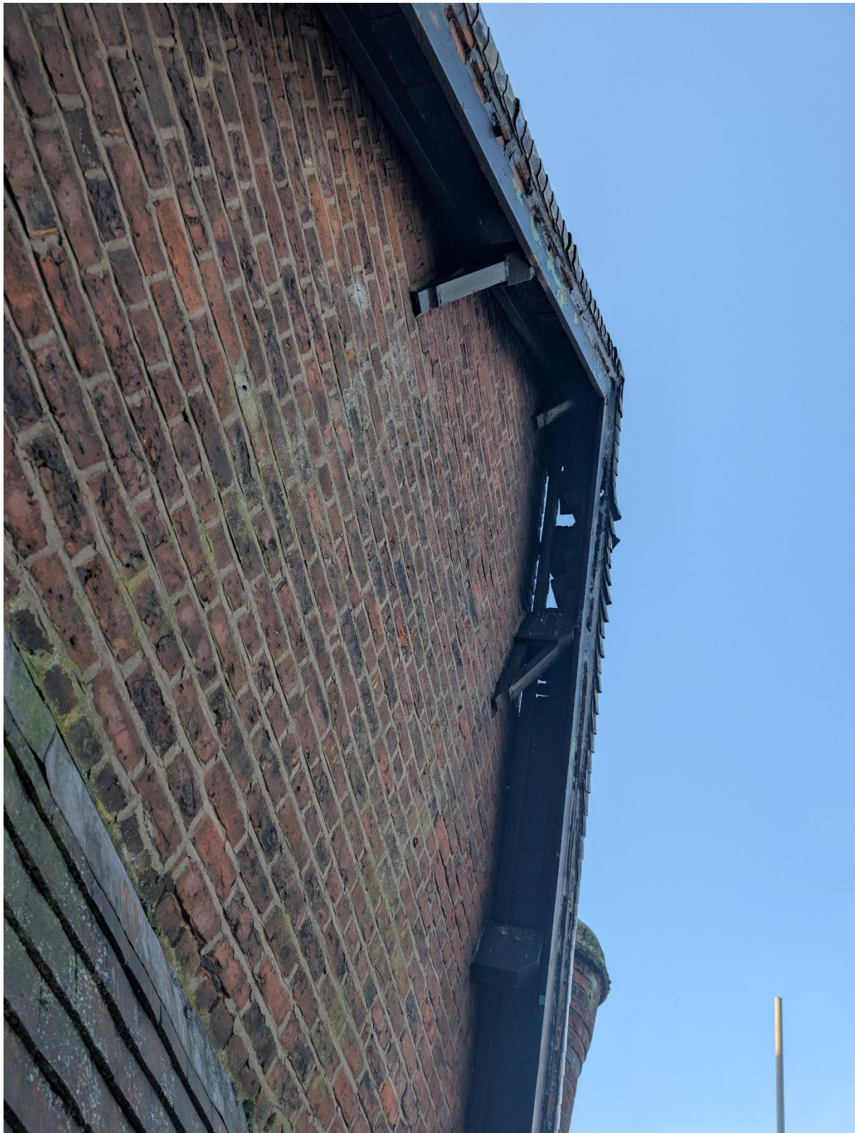
Picture 12 Rear Roof Overhang
