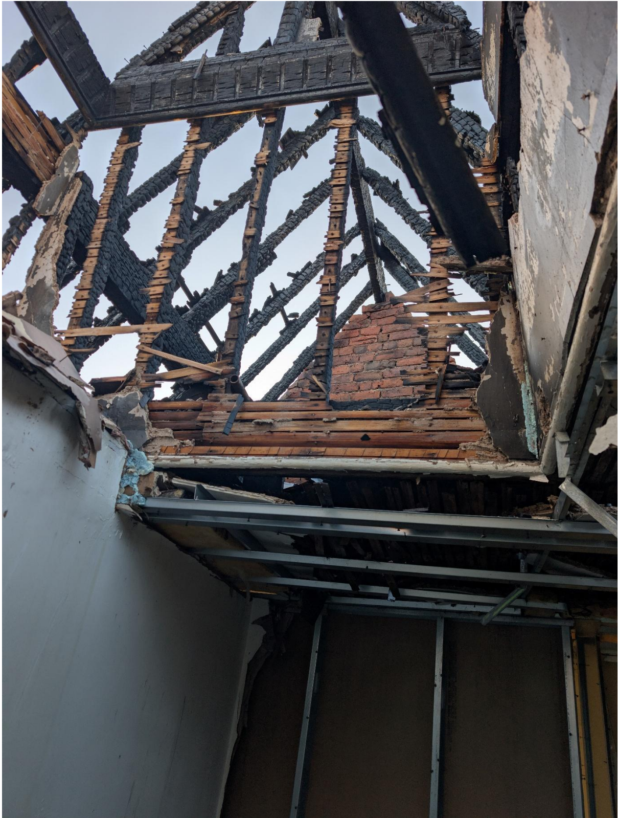
Picture 15 View In Roof From 4th Floor
