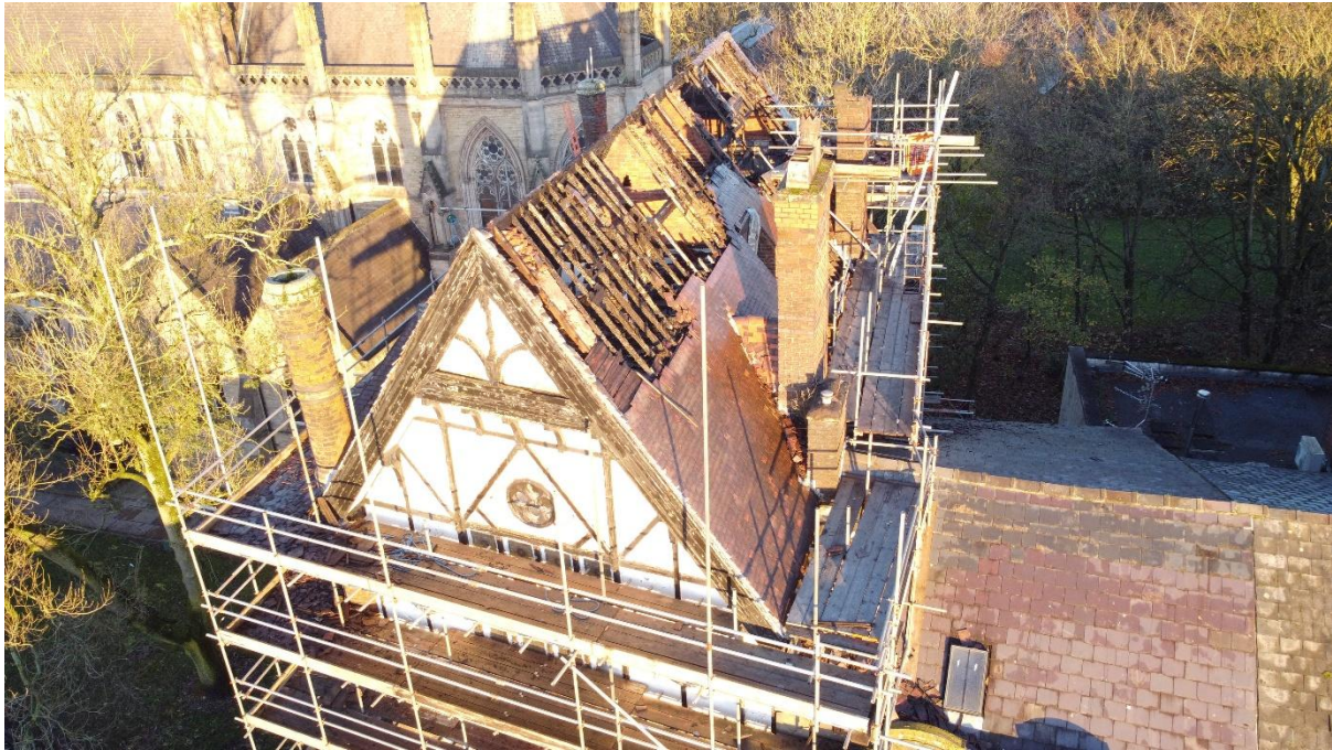
Picture 1 View On Roof
