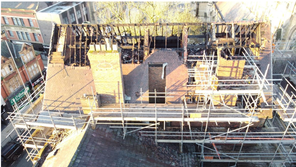
Picture 2 View On Roof
