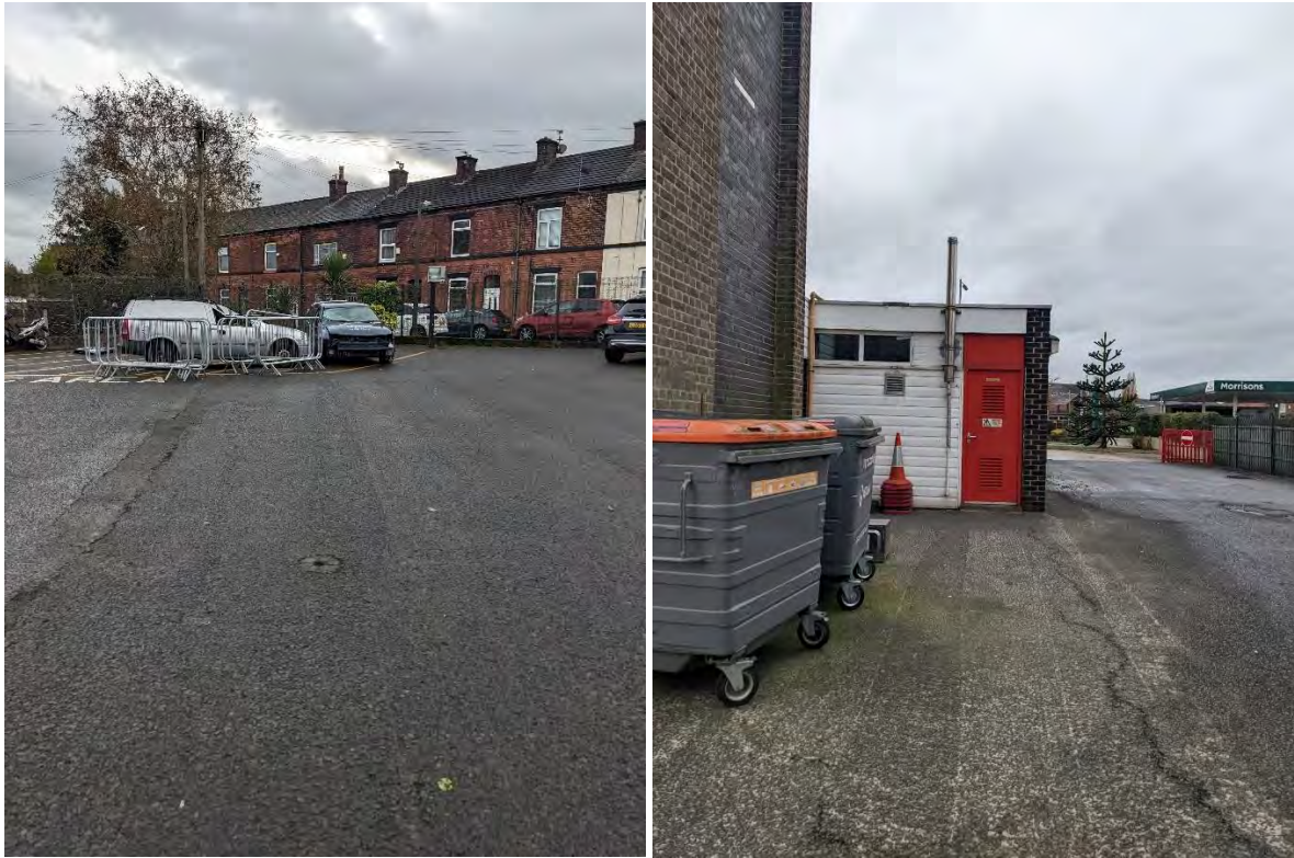
Figure 5: Photographs of the vehicles and boiler room
