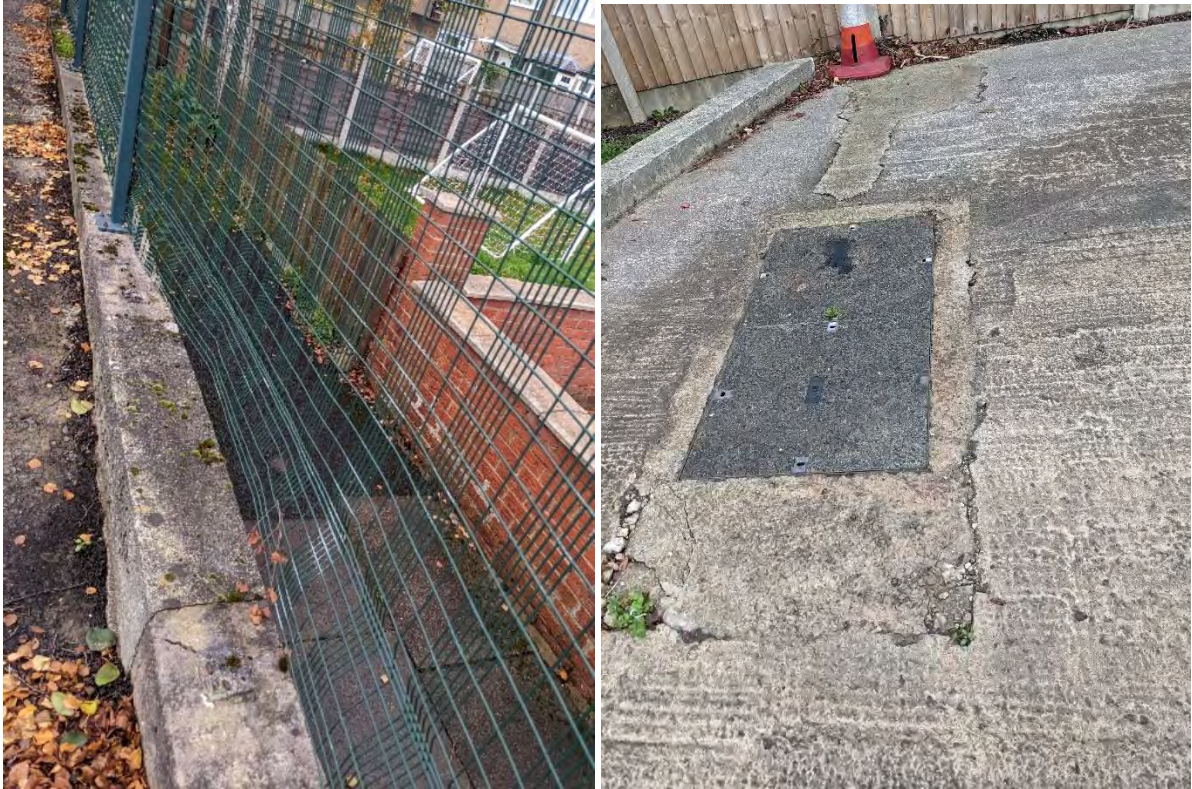
Figure 3: Photograph of the retaining wall (left) and service manholes (right)
