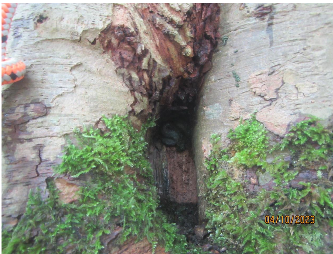
Photograph 2 – The superficial stem cavity at approximately 4m.
