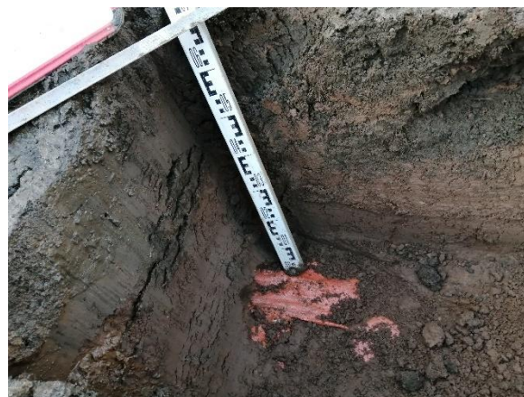
Evidence of Warning Membrane
