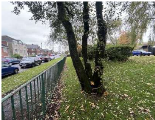
Photo 17 - Low-level iron railings to the front boundary adjacent to the main road, which do not provide an effective safeguarding barrier or meet current DfE requirements for secure school perimeters.
