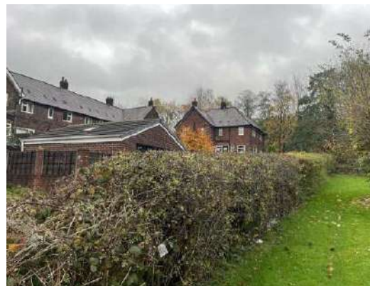
Photo 6 - Unmanaged vegetation obscuring boundary fencing, concealing access points and compromising safeguarding and visibility on the north boundary.
