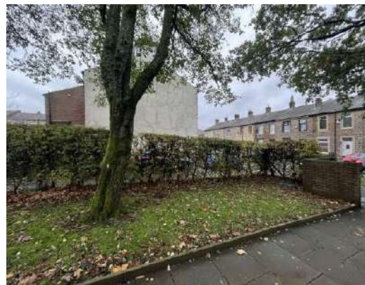
Photo 16 - Front boundary reliant solely on hedging, with no physical fencing and unrestricted public access to the school site.
