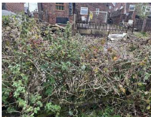
Photo 5 - Vegetation growth provides climbing assistance, enabling unauthorised access over the boundary and undermining perimeter security on the north boundary.
