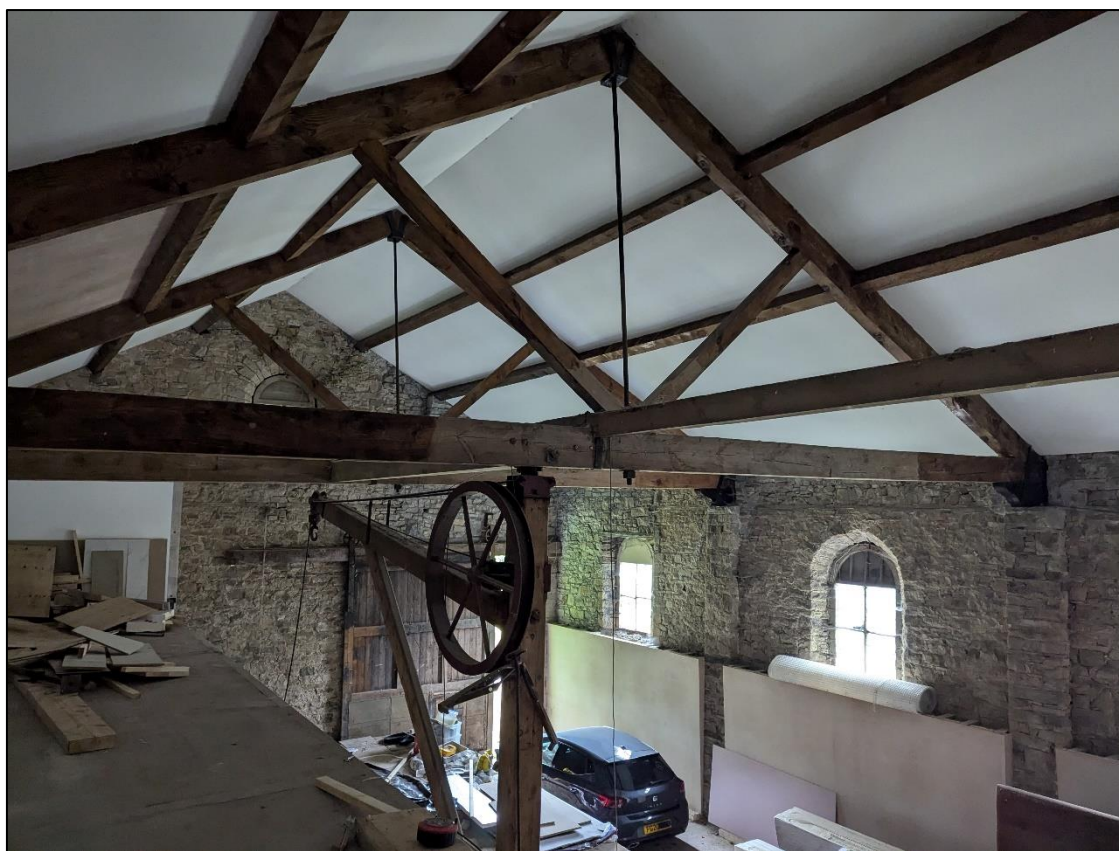
Plate 30: Truss and crane from mezzanine
