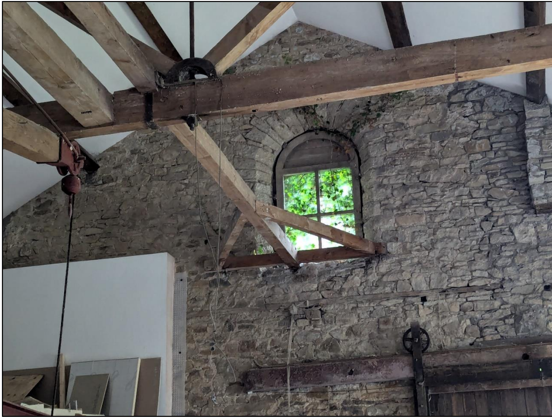
Plate 23: Braced beam spanning the room
