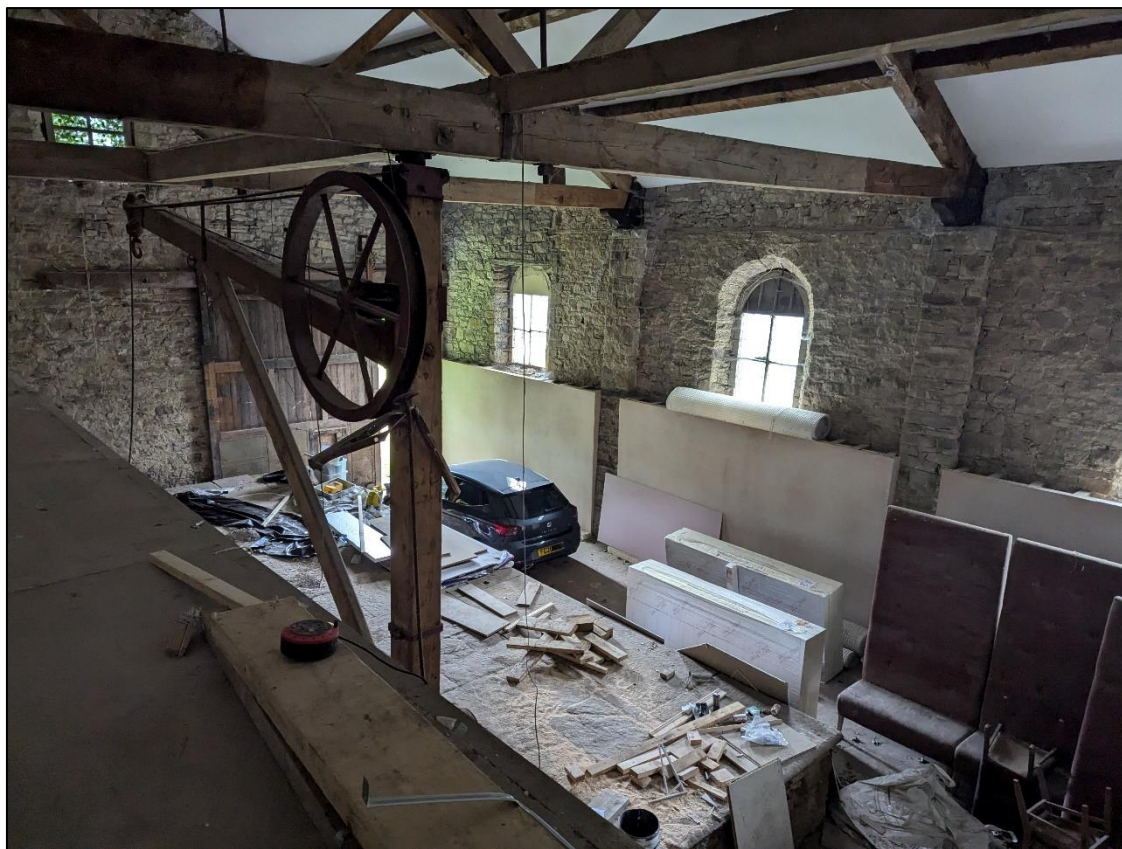
Plate 32: General view of interior from mezzanine looking south
