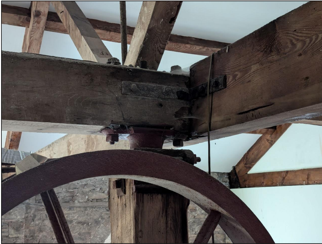
Plate 21: Crane fixing to beam
