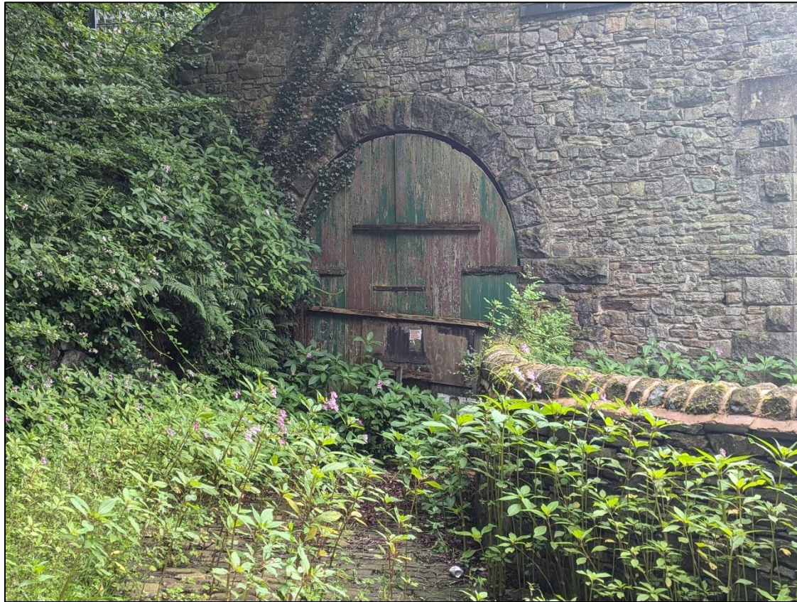
Plate 11: Road vehicle loading doorway
