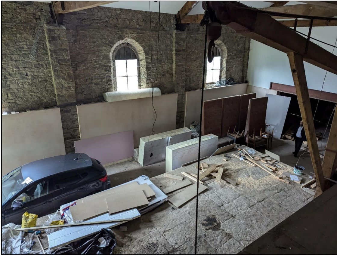
Plate 33: General view of interior from mezzanine looking north
