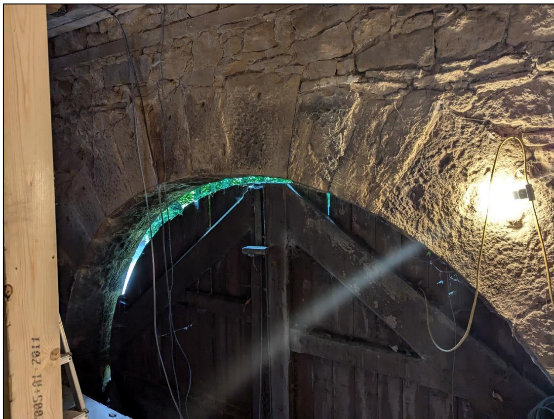
Plate 28: Detail of interior stonework of arched lintel of road traffic loading door
