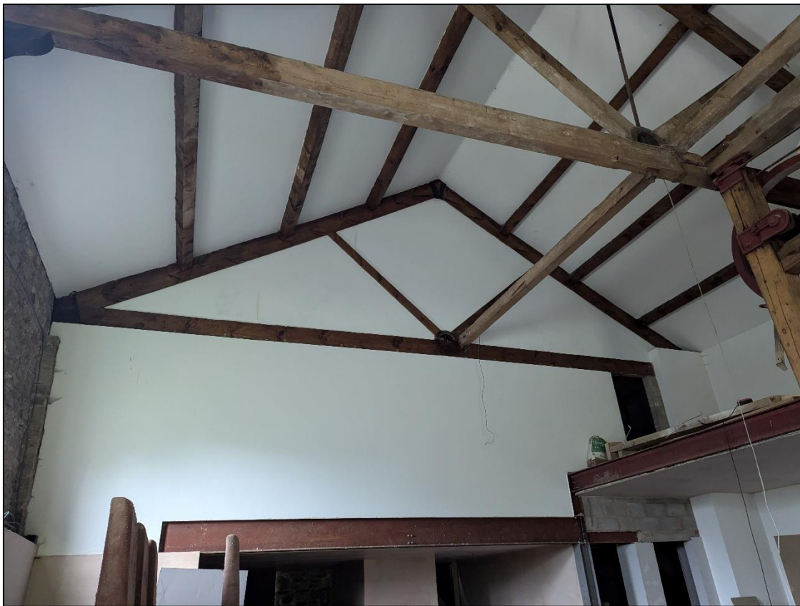
Plate 26: Inserted wall to northern end
