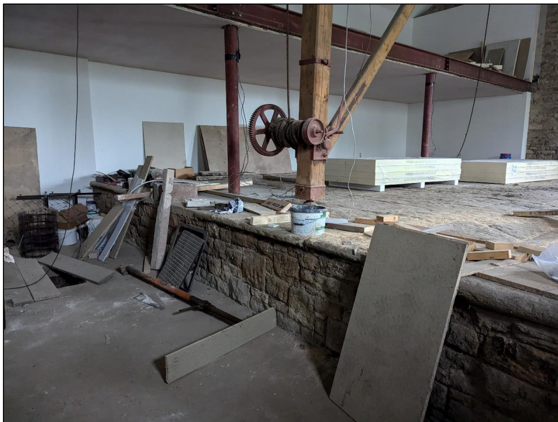
Plate 16: Loading platform and crane
