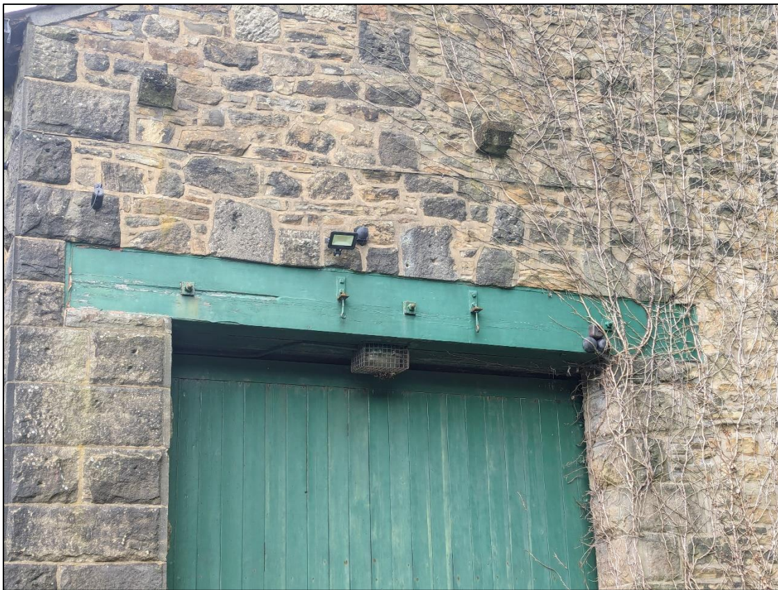
Plate 4: Detail of timber lintel
