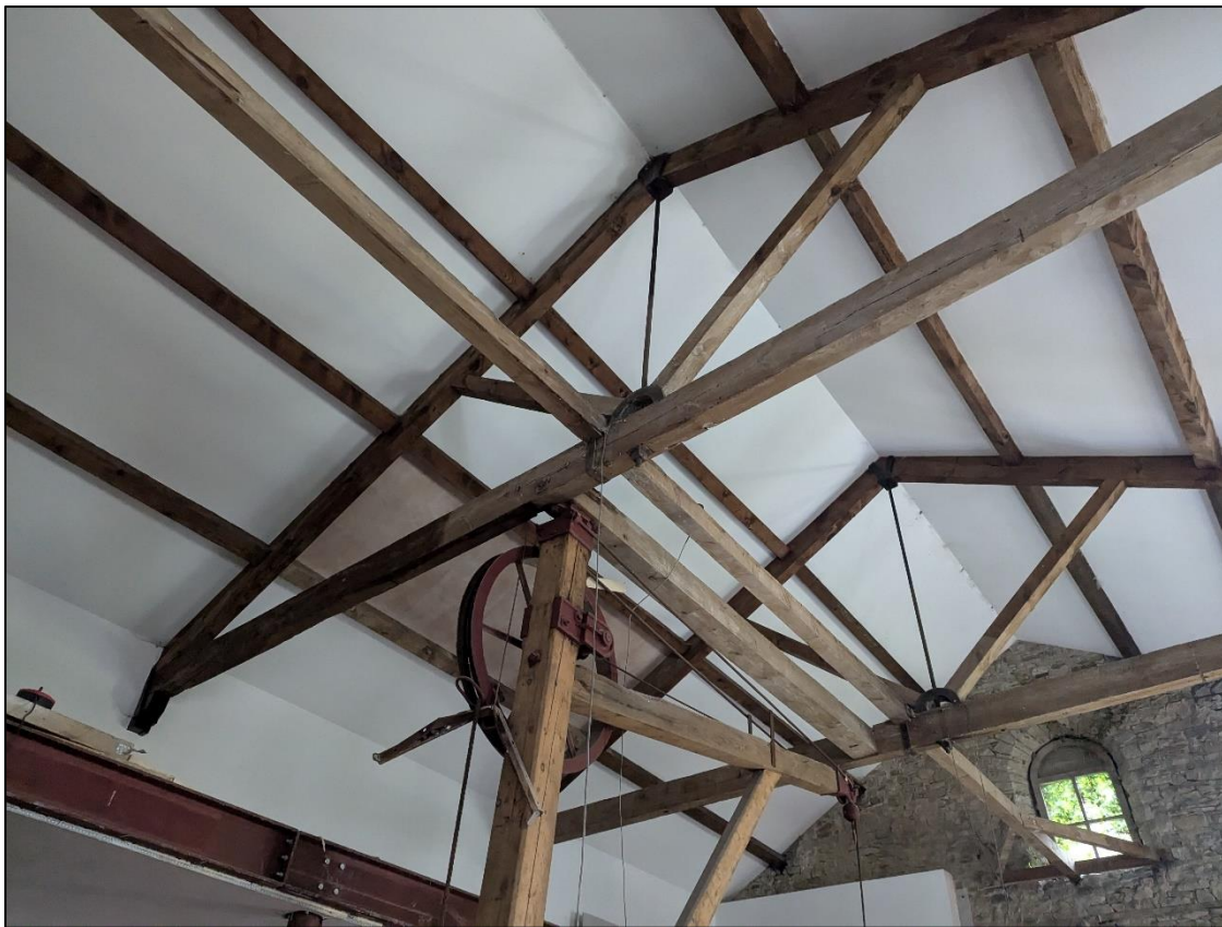
Plate 24: Crane in relation to truss
