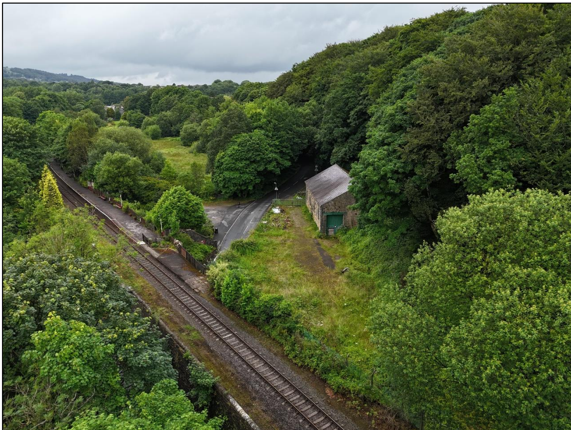
Plate 34: View of shed in relation to railway
