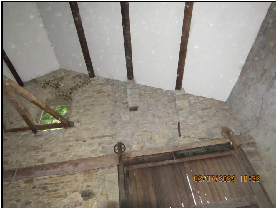
022 Upper pike, South West gable
