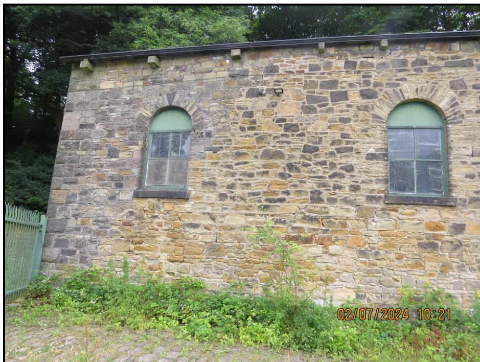
010 Western flank, 0 – 9 metres
