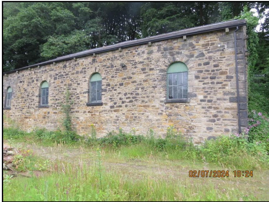
Photograph 012 Western flank, 0 – 20 metres
