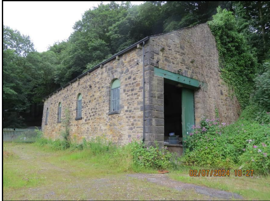
Photograph 014 Western flank and Southern gable
