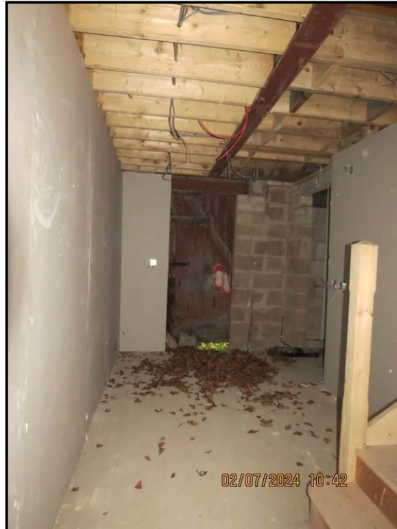
044 Stairs to first floor
