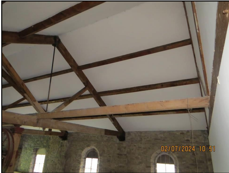
057 Western roof slope
