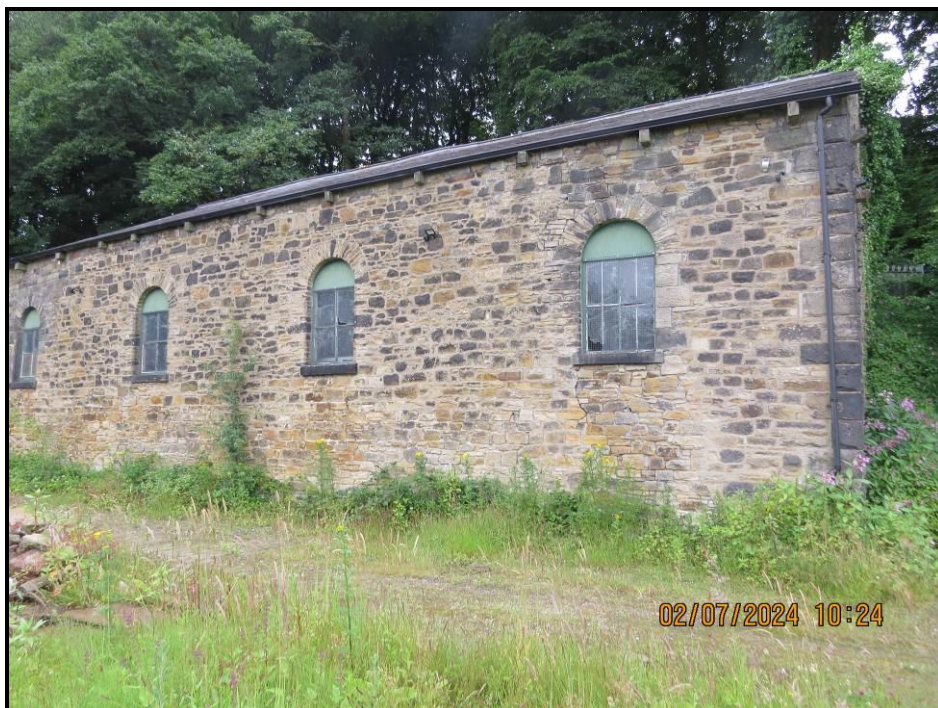
012 Western flank, 0 – 20 metres
