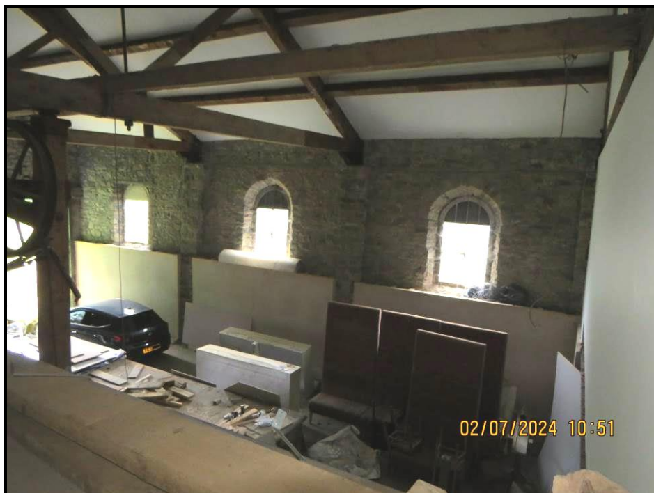
056 Western elevation, windows 4 – 2
