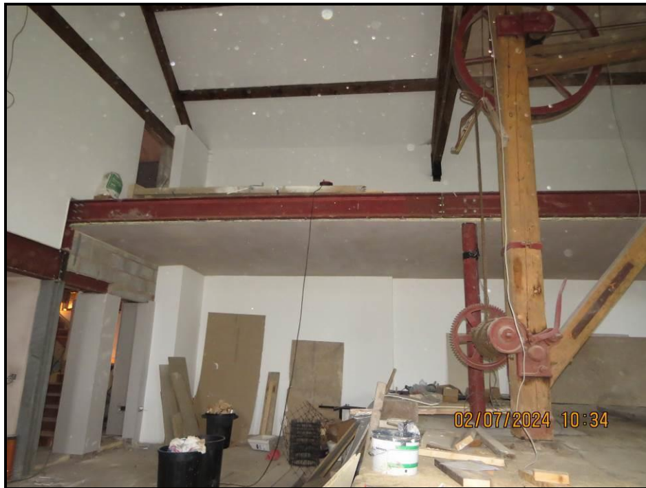
024 Eastern flank, chainage 5 – 10 metres
