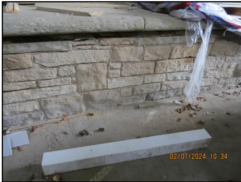
Photograph 027 Typical plinth construction
