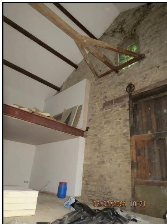
019 Southern gable (South East)
