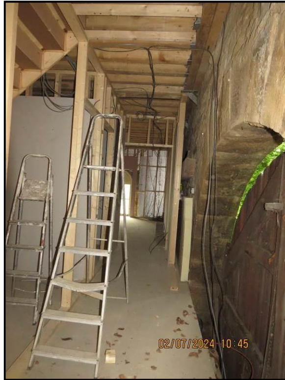
046 North Eastern arch
