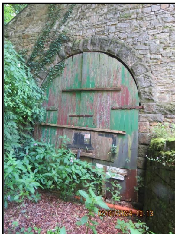
004 North Eastern arch
