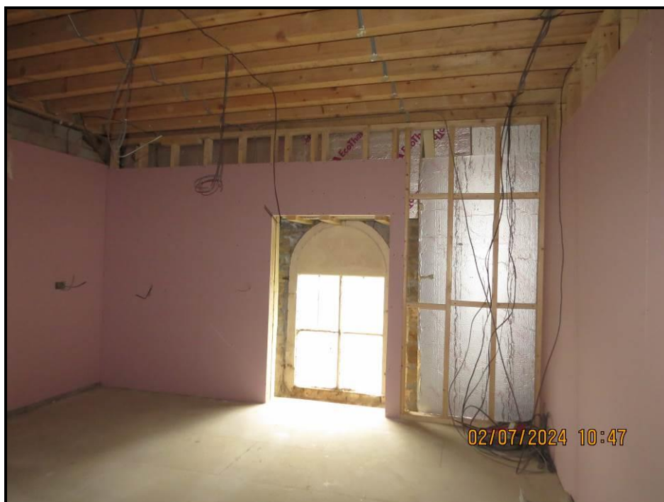
051 Mid floor level, North West corner
