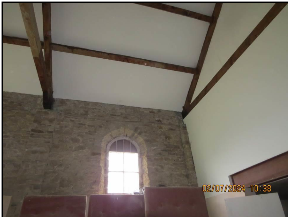
035 South West corner, Trusses 2 and 1
