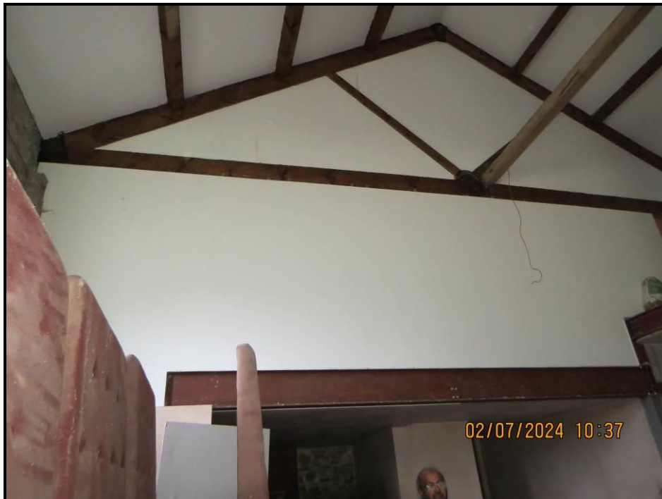
032 Truss 1, chainage 5 metres
