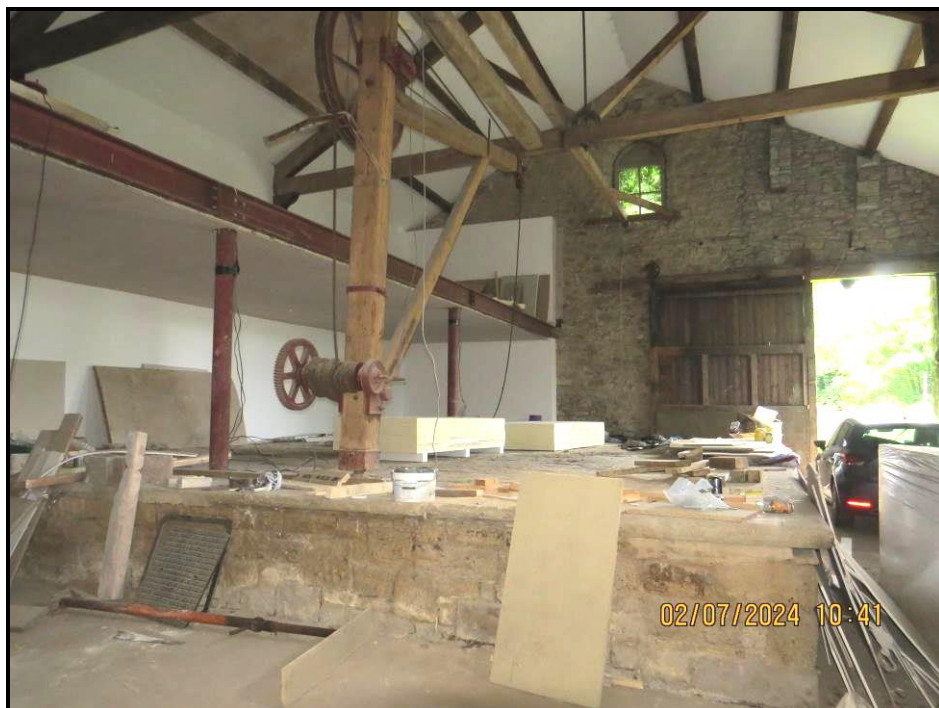
043 Eastern flank and Southern gable
