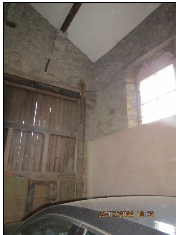
023 Southern gable and Western flank
