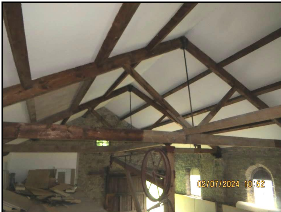
058 Satisfactory truss bearing
