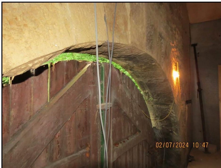
048 North Eastern arch internal profile
