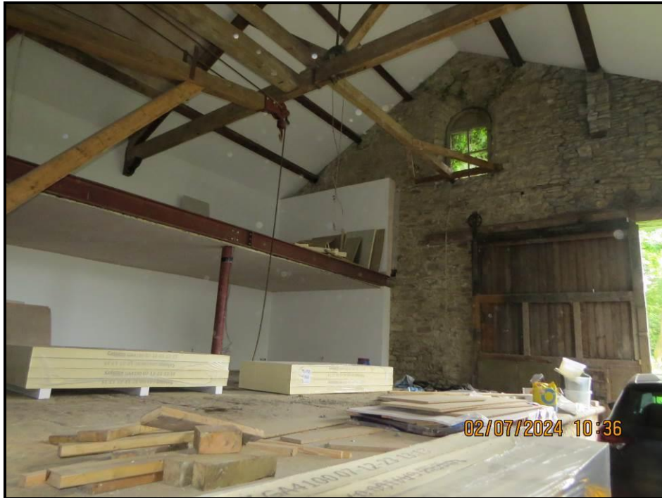
028 Southern gable (South East)
