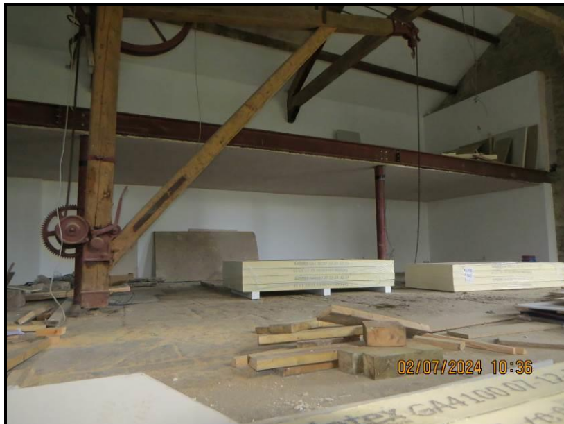
Photograph 030 Crane and loading platform
