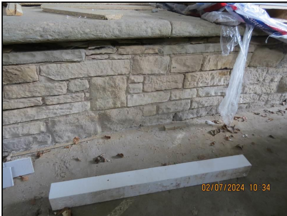
027 Typical plinth construction
