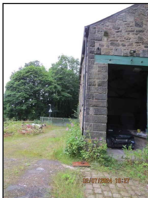
015 Good vertical alignment to Western flank
