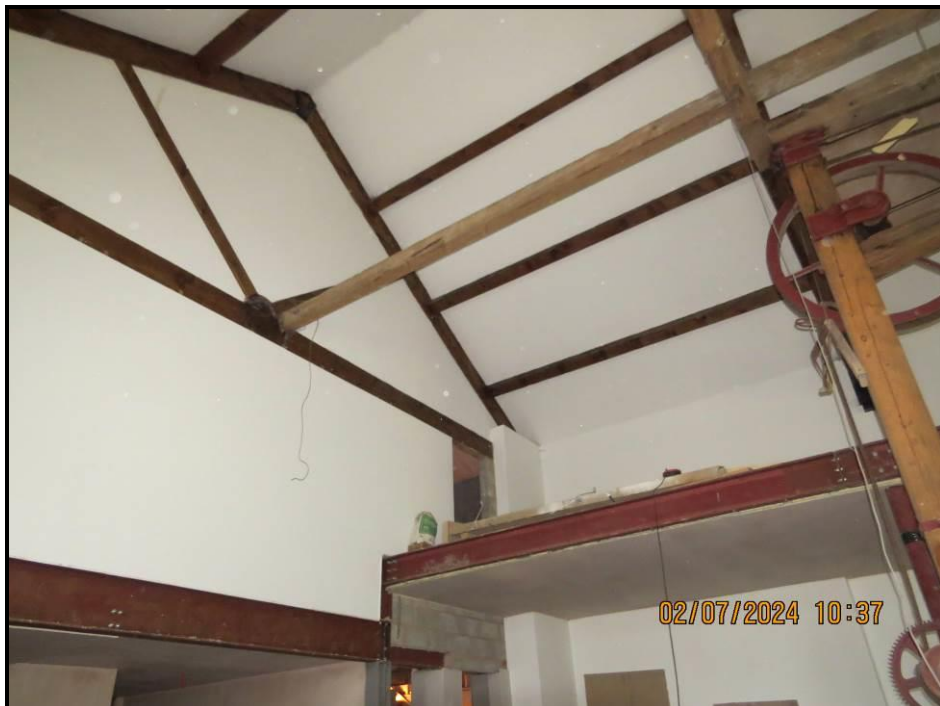
031 North Eastern truss 1 – 2
