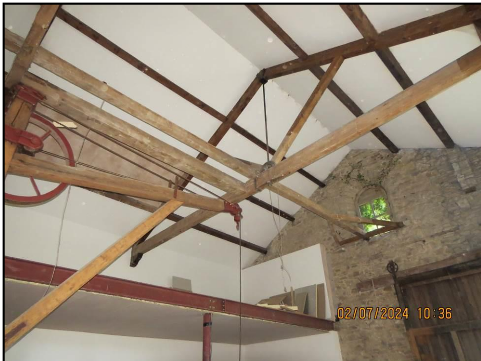
029 Truss 3 (South East)
