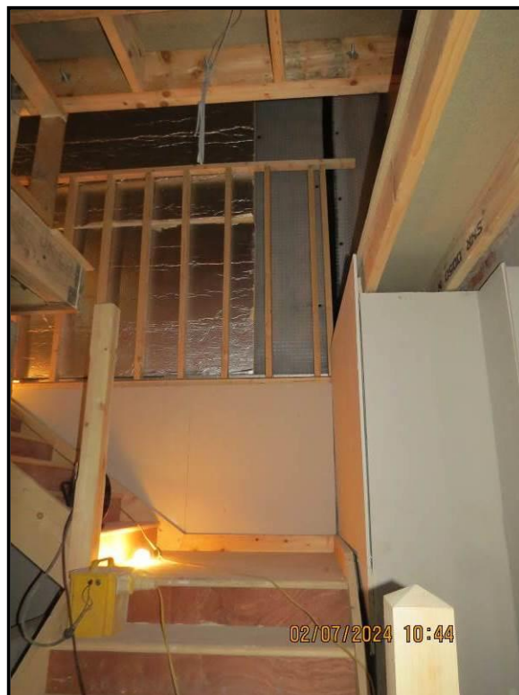
045 Stairs to first floor
