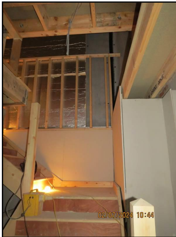
Photograph 045 Stairs to first floor
