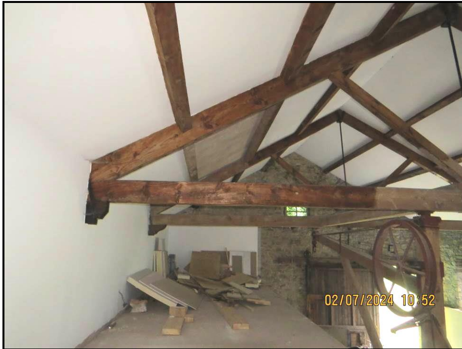
059 Satisfactory truss bearing
