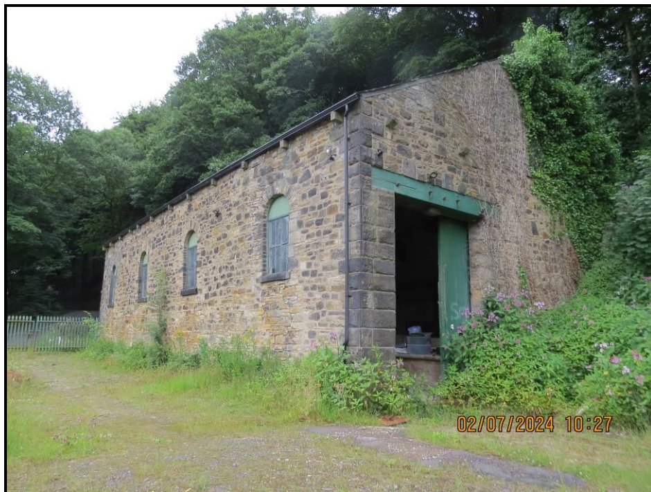
Photograph 014 Western flank and Southern gable
