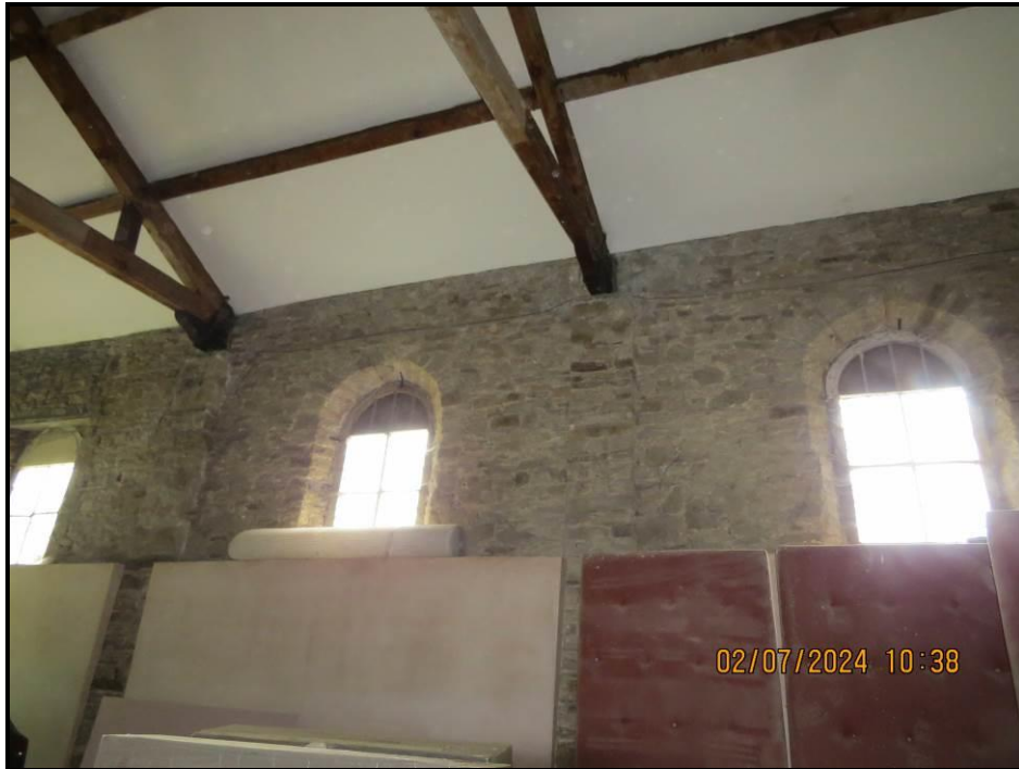
034 Western flank, trusses 2 and 1
