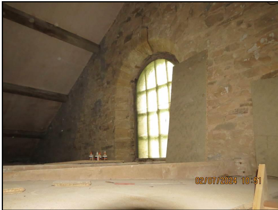
055 Upper floor, North Western gable
