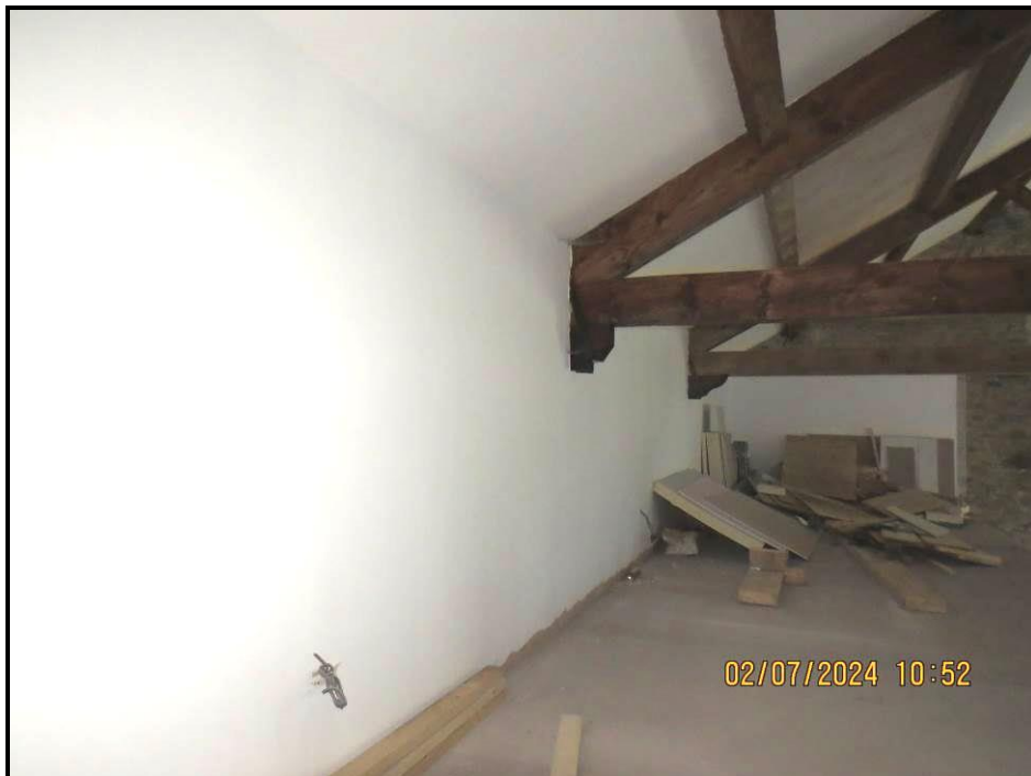
060 Satisfactory truss bearing
