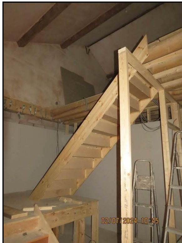
047 Stairs to upper floor
