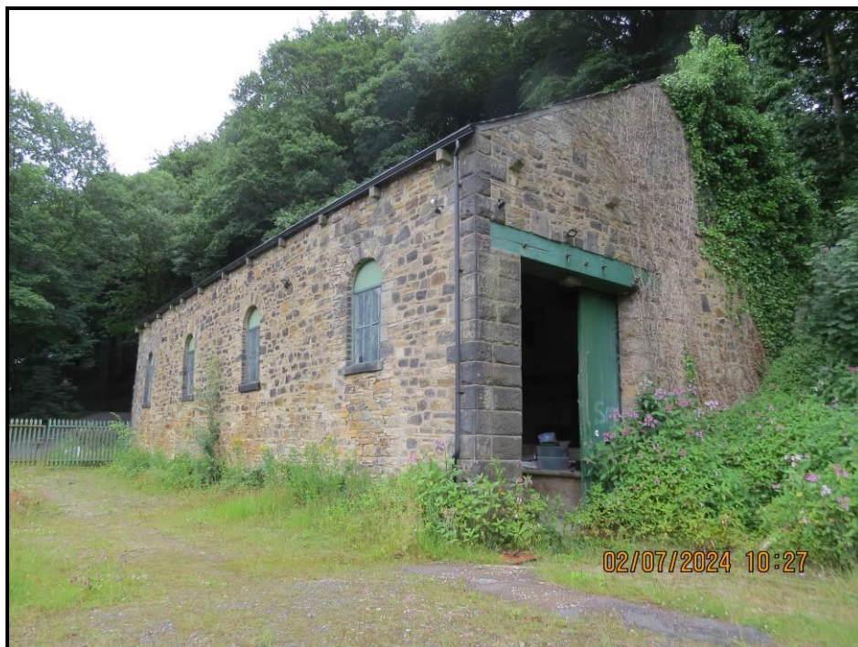
013 Western flank, 7 – 20 metres
