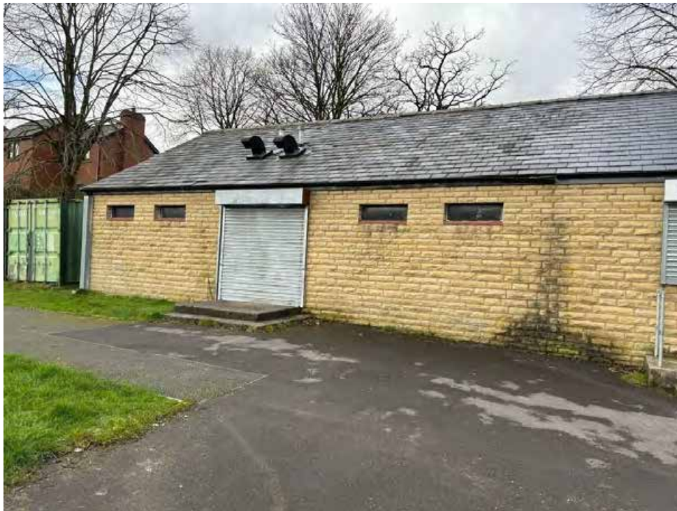
Figure 1: A photo of the existing pavilion on site.
