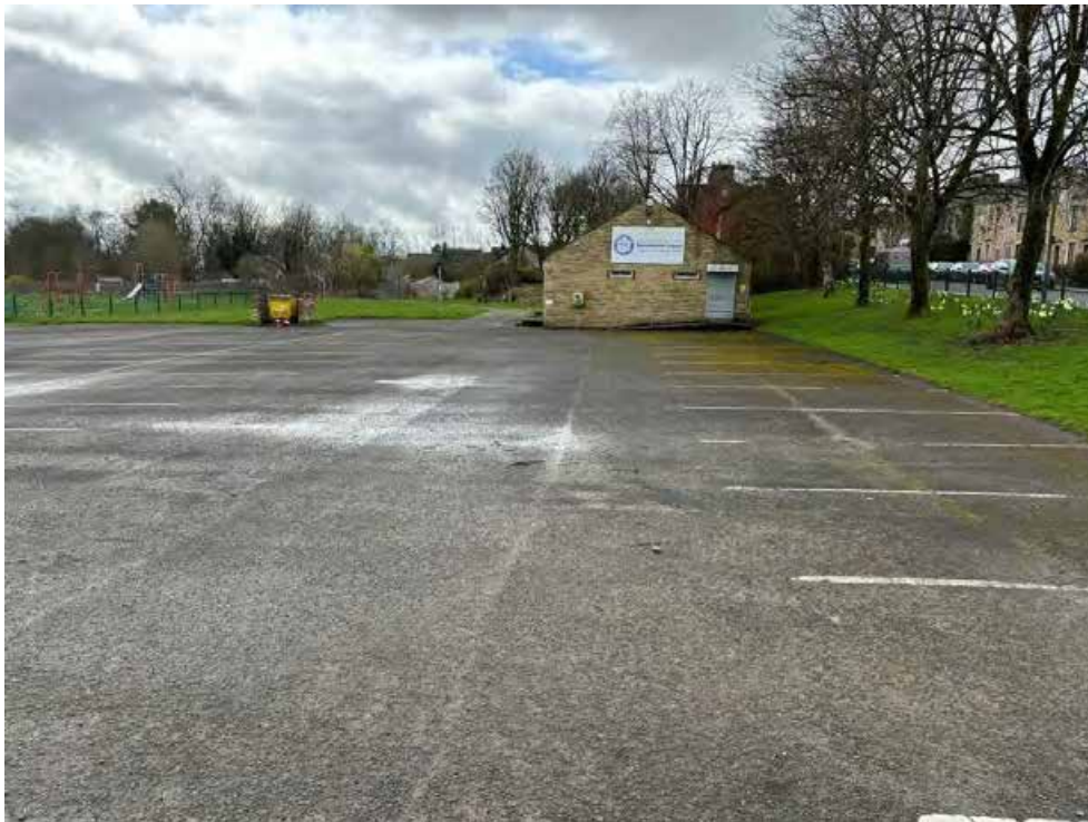
Figure 3: A photo of the carpark on site.
