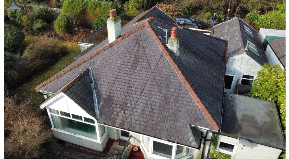
B1 – eastern roof structure
