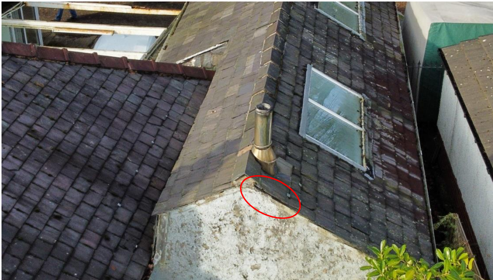
B1 – roof of garage/outbuilding section
