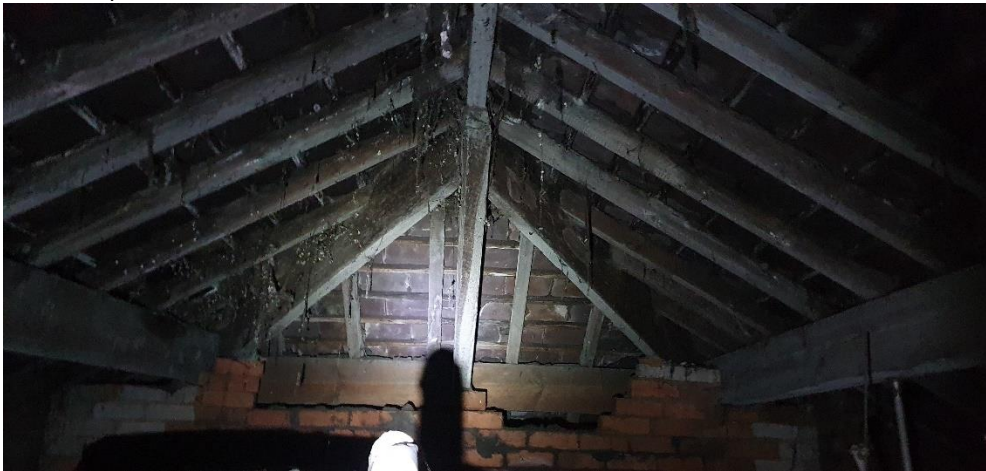
B1 - loft interior looking east
