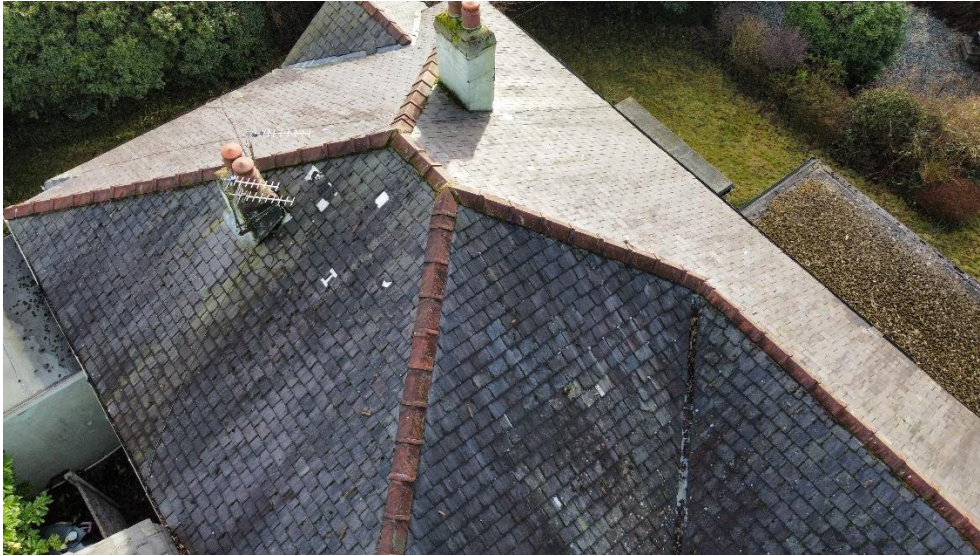
B1 – central roof structure
