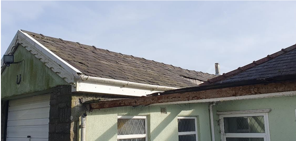
B1 – southern elevation of garage/outbuilding
