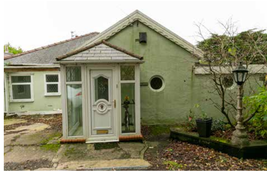
EXISTING FRONT ENTRANCE PORCH
