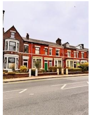
Figure 2.4: View of application property and neighbouring properties from Walmersley Road
