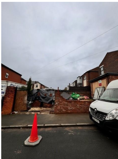
Figure 2.9: View of application property and neighbouring properties from Clifton Road
