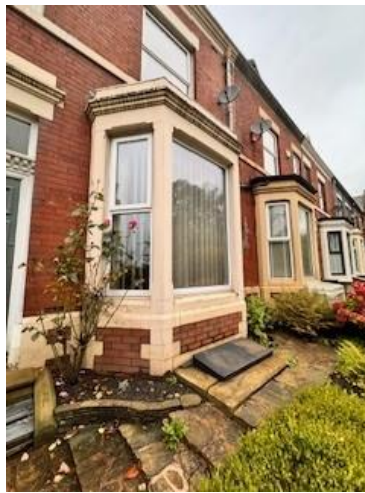
Figure 2.3: Bay window and existing lightwell
