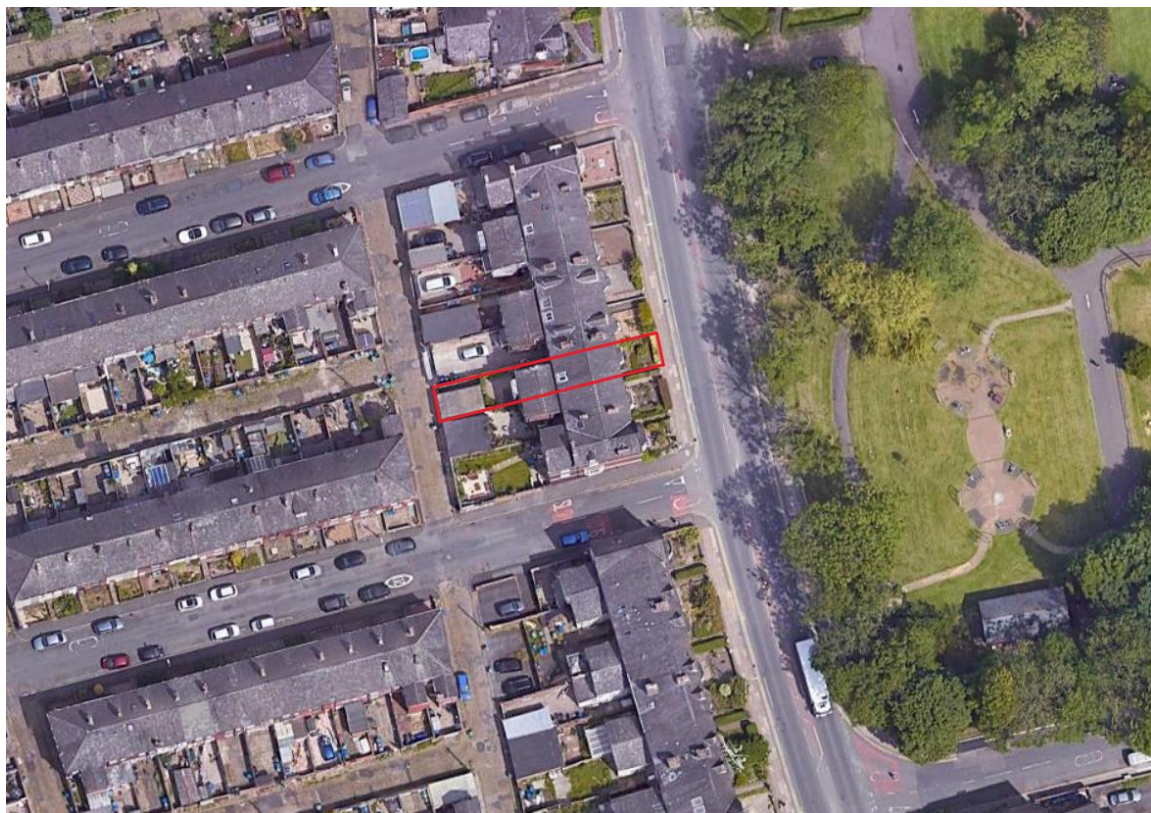
Figure 2.1: Aerial view of application site (outlined in red)
