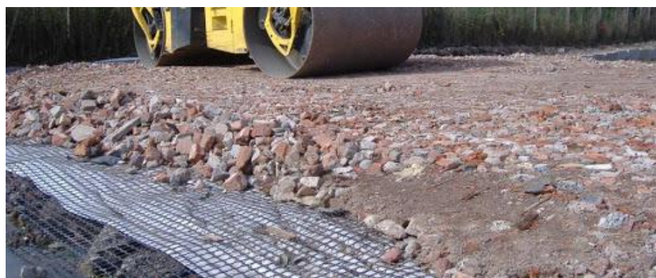
Intsalation of hardcore (crushed brick) and compaction of the same, the geotex is then used to bind the layers together.
