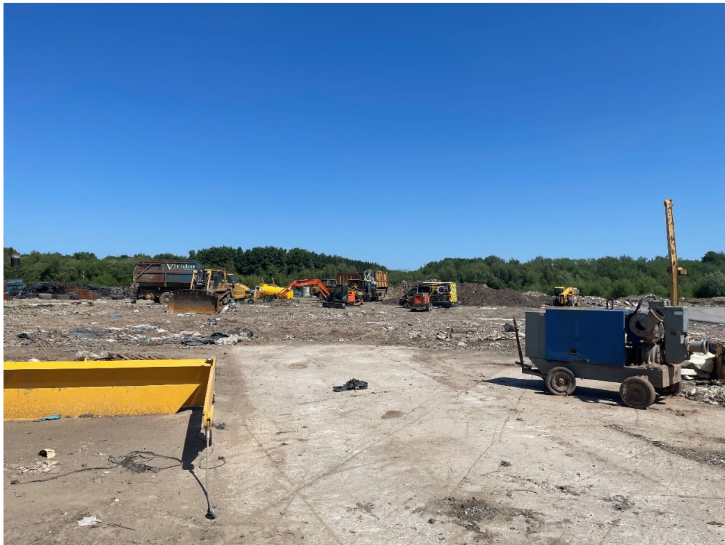
Image 2 of Site from within Pilsworth South Landfill
