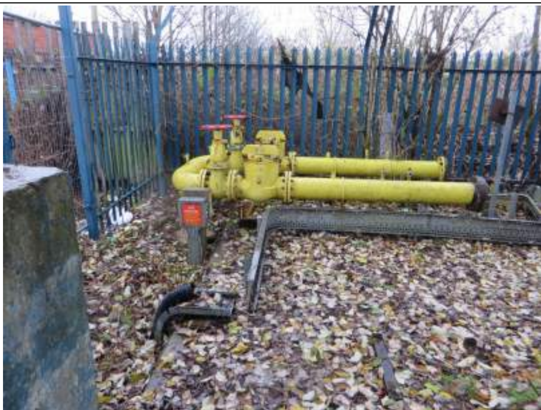
Photo 12: Onsite utilities were identified across the site including gas pipeline located towards the eastern boundary.
