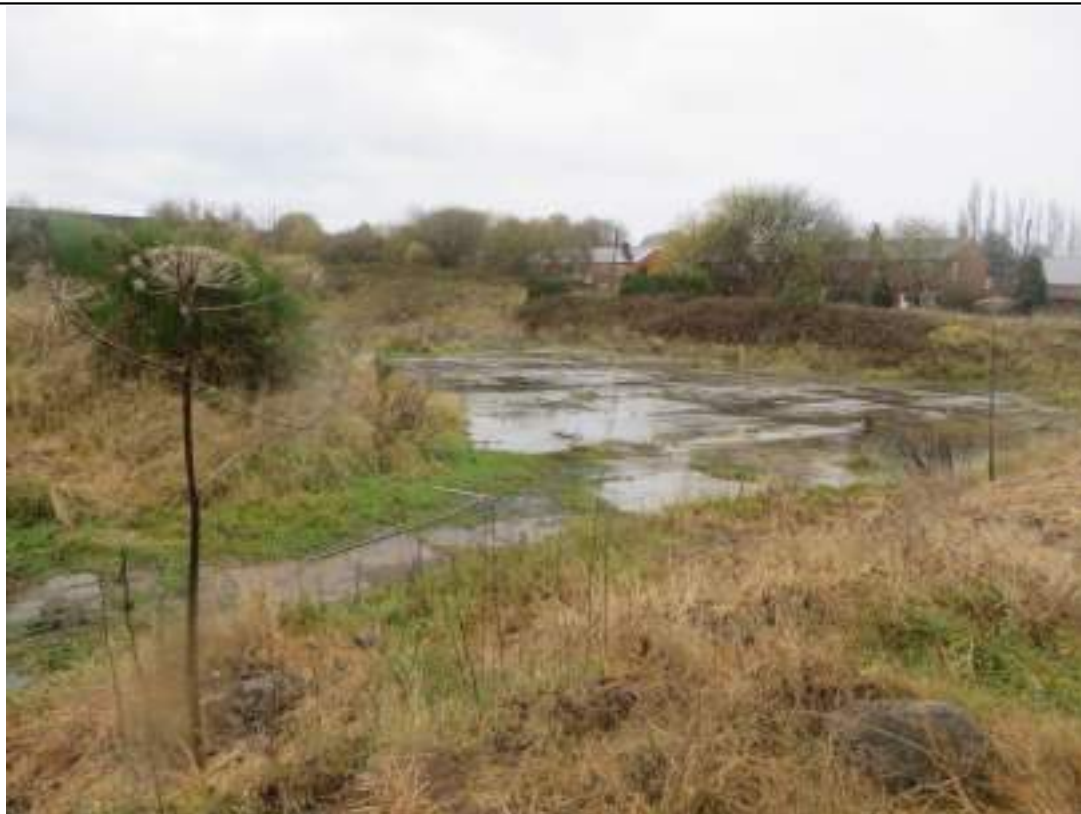
Photo 13: Concrete hard standing associated with a former mill towards the southwest of the site.
