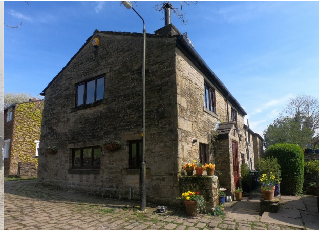
West and south elevations
