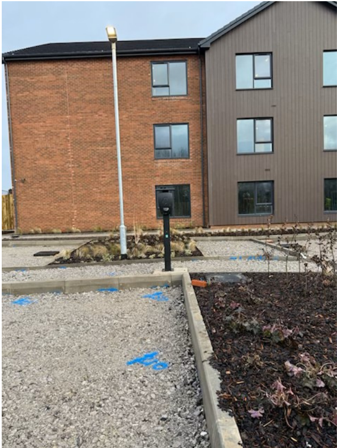
Photographic evidence of the installation of the EV Chargers
