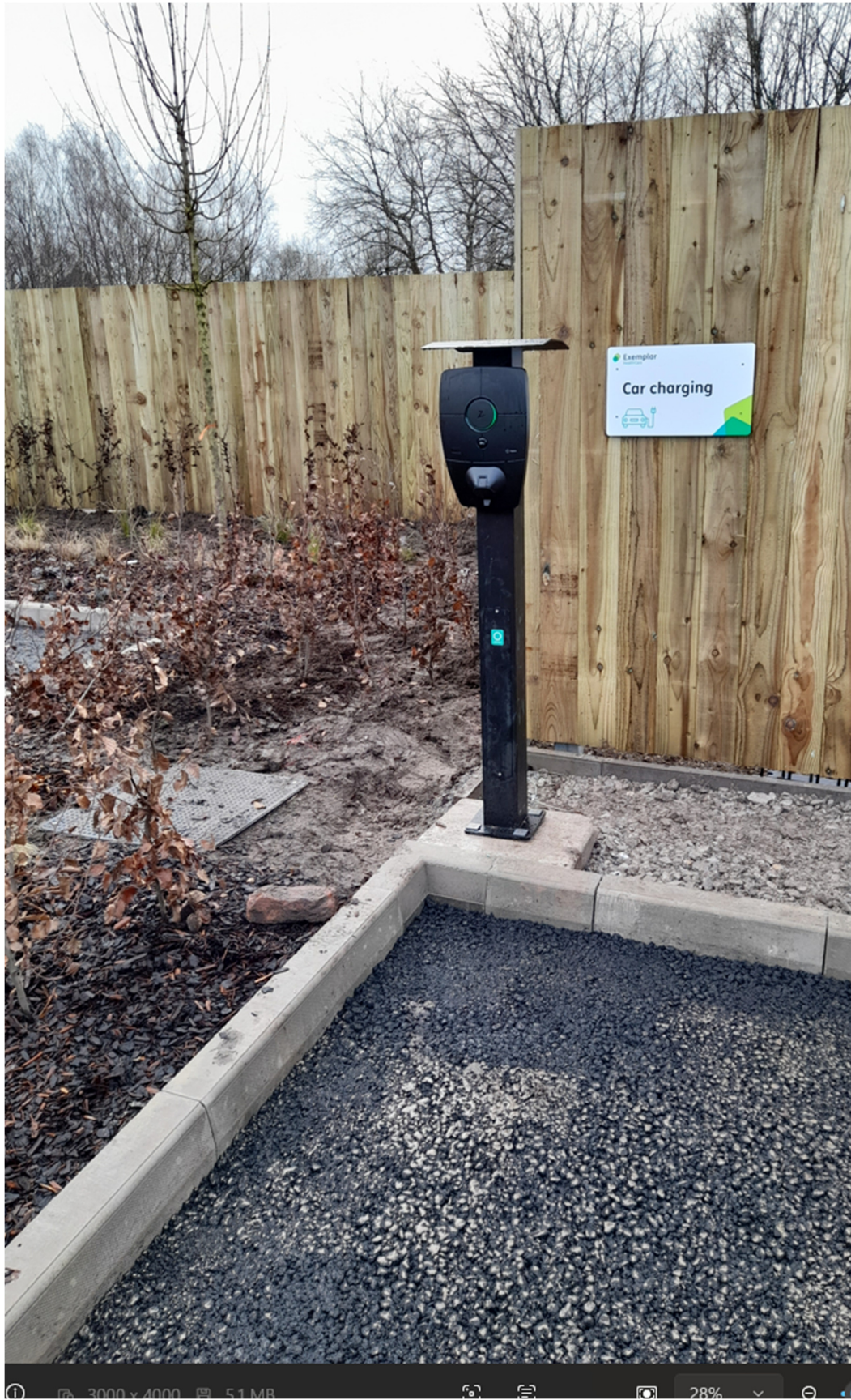
Photographic evidence of the installation of the EV Charger to Parking Bay 1
