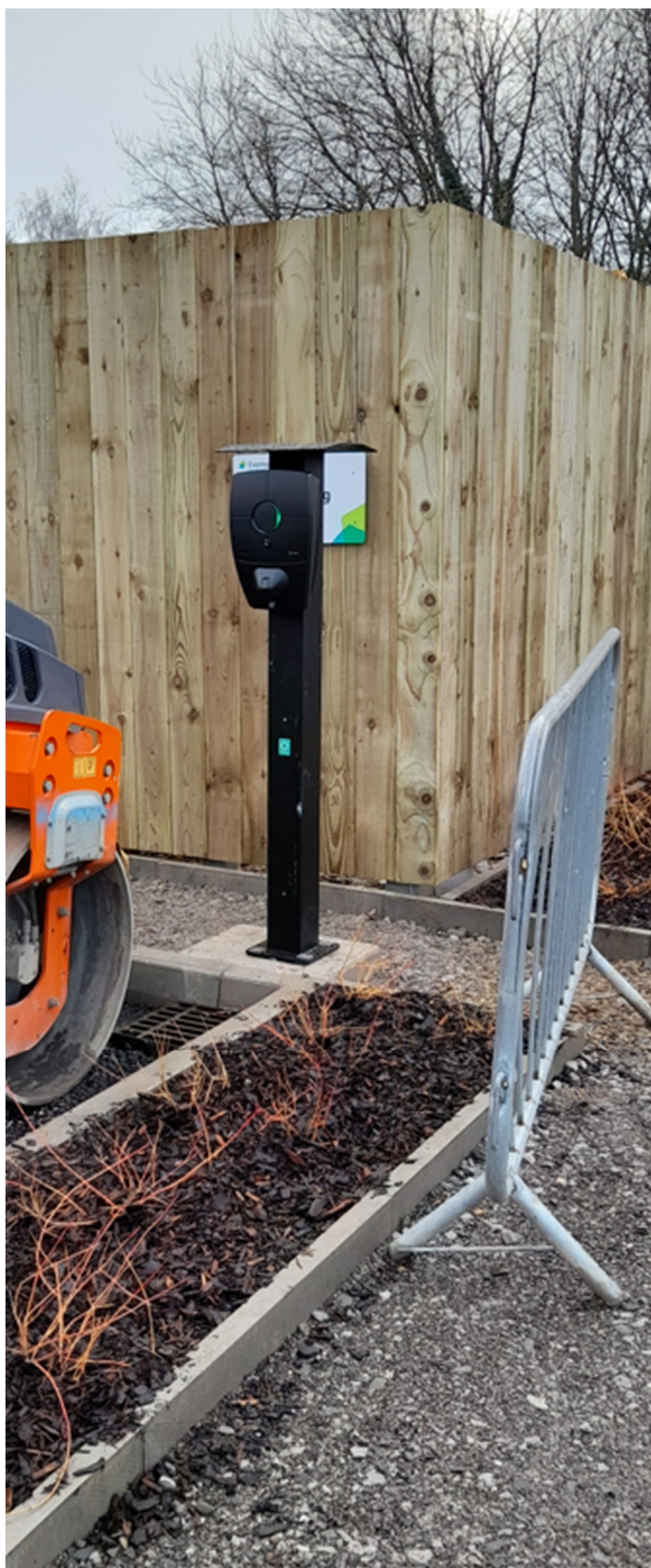
Photographic evidence of the installation of the EV Charger to Parking Bay 2
