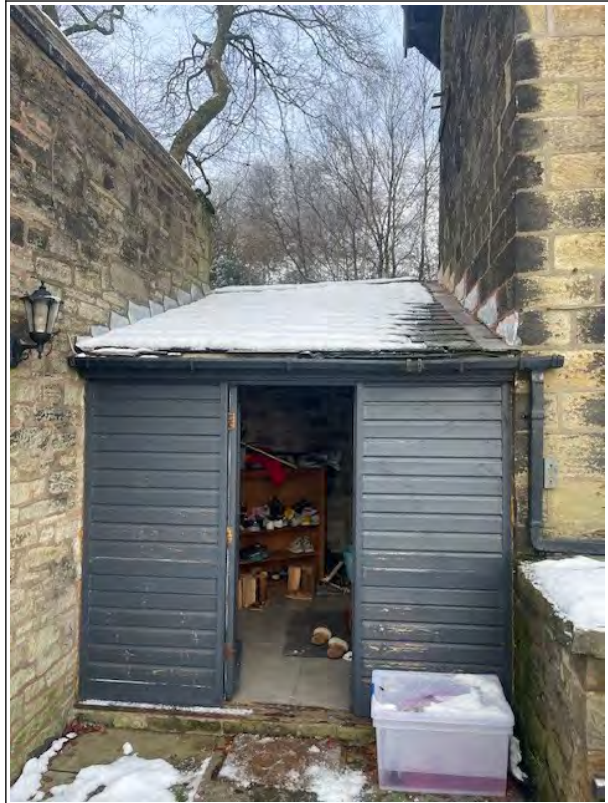
Photo 2: Front of timber porch proposed for replacement
