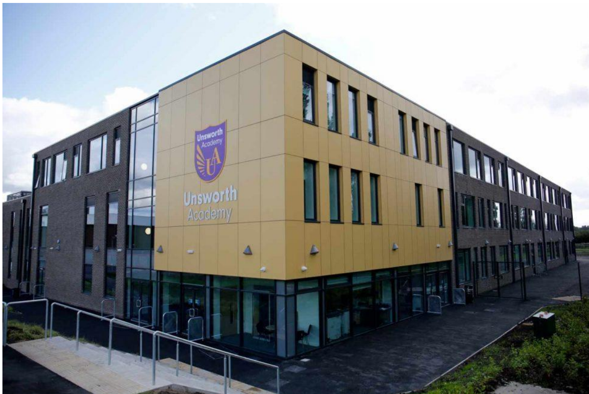
Image . Existing school building
