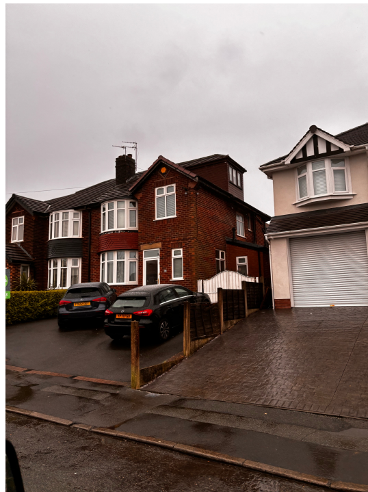
Contemporary Extensions and finishes to Front Elevation
