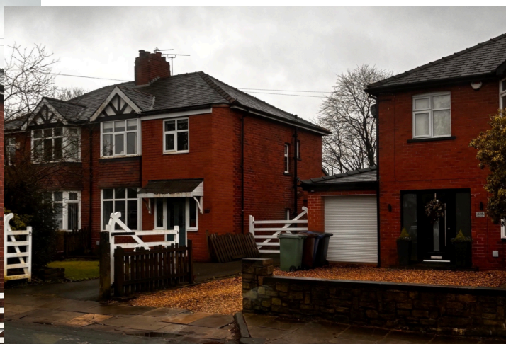
Double height front (infill extension squaring off - flat roof).
