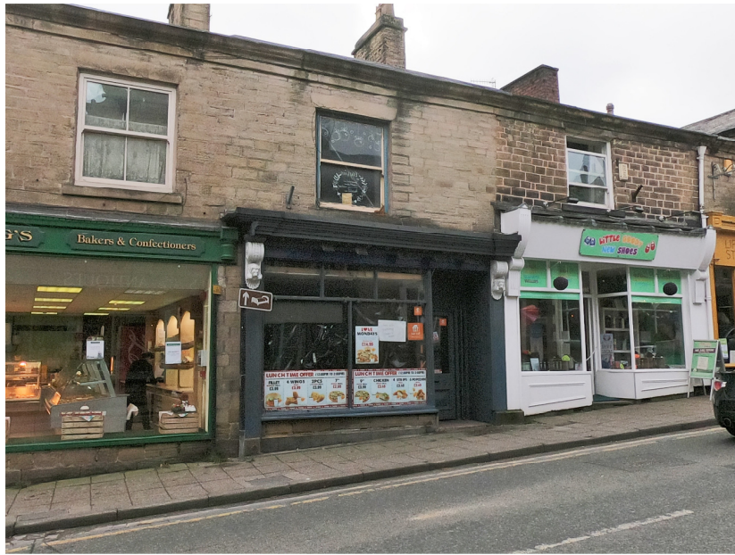
Well preserved Victorian timber shop front
