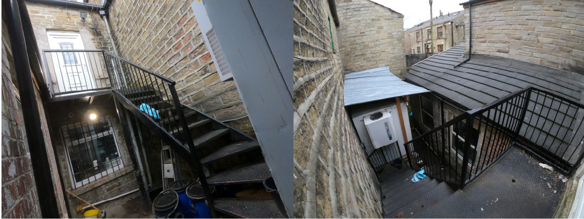
Stairs in the rear yard
