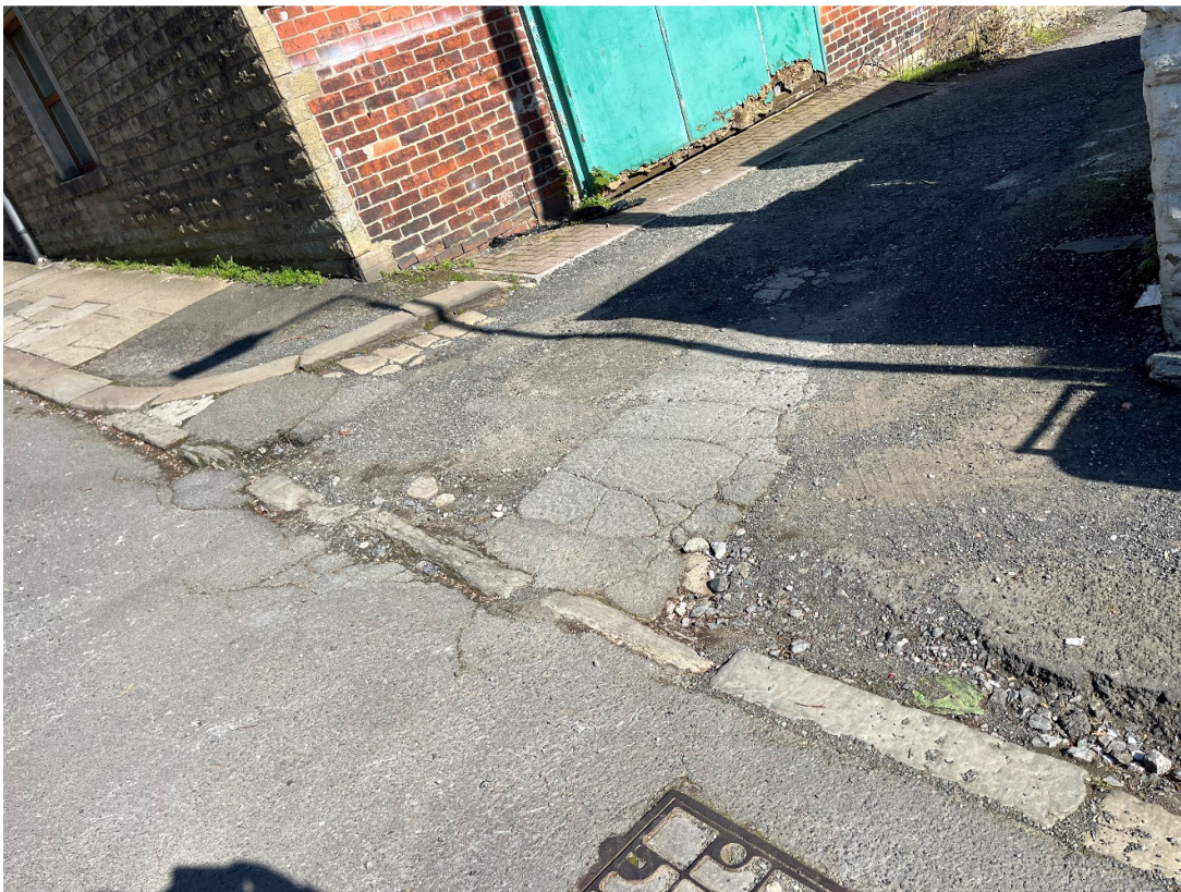
7. Road edge Spring Street meets Caltha Street
