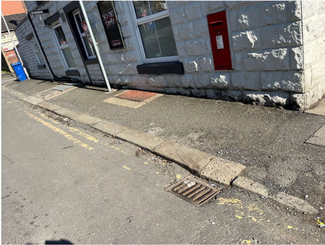
4. Pavement along Spring Street adjacent The Major P.H.
