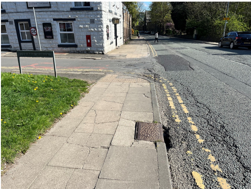
1. Pavement looking along Bolton Street towards Ramsbottom town centre
