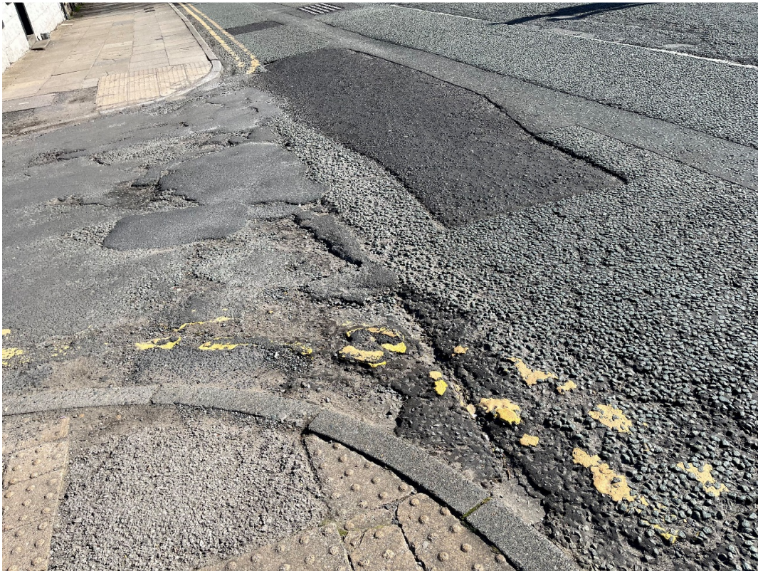
2. Tarmac along the junction of Spring Street and Bolton Street
