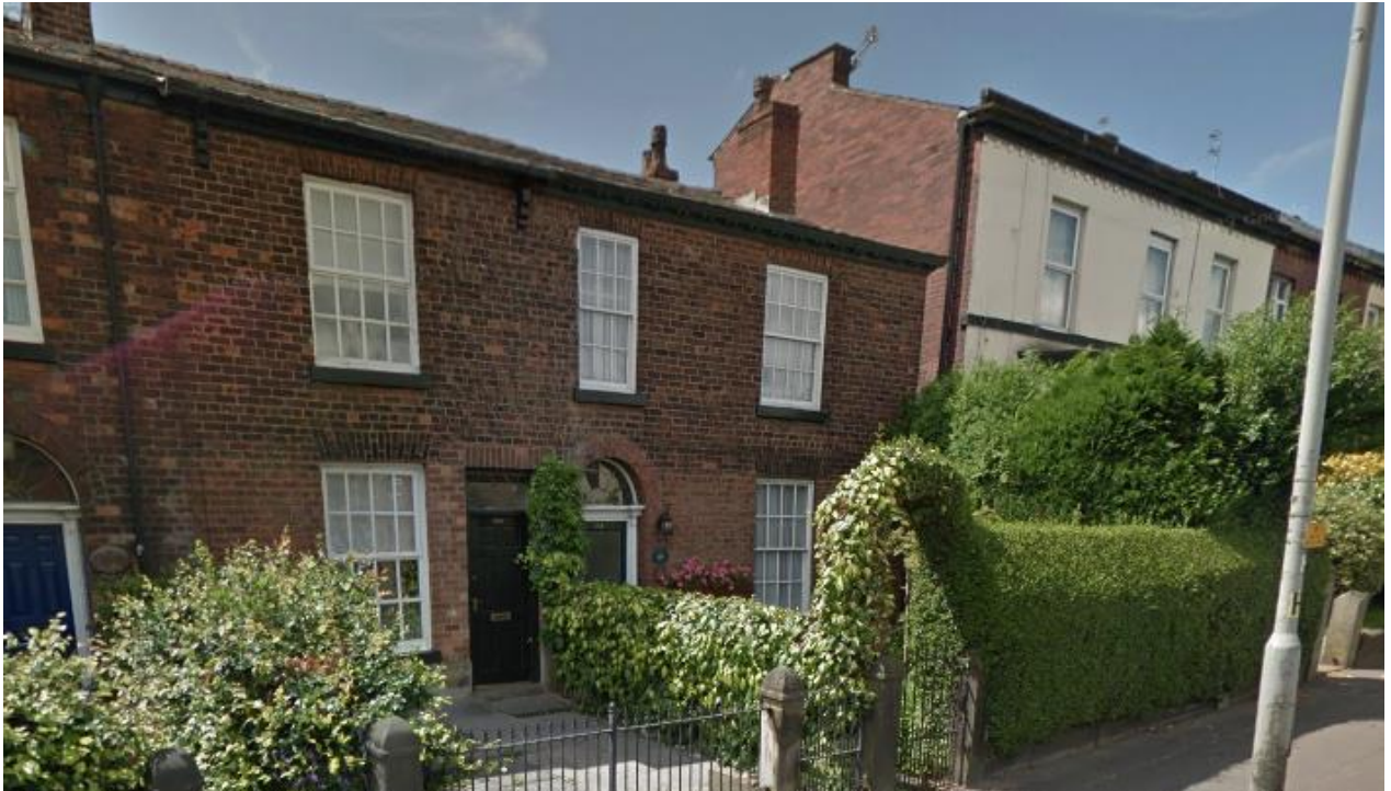
Fig 5. Front elevation of 108 (right) and 108A (left) taken from Google Streetview circa 2017
