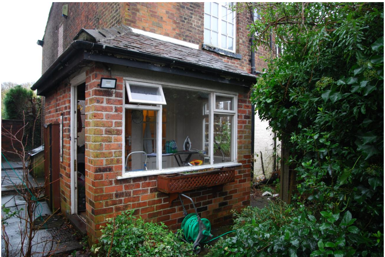
Fig 7. Existing rear single storey extension.
