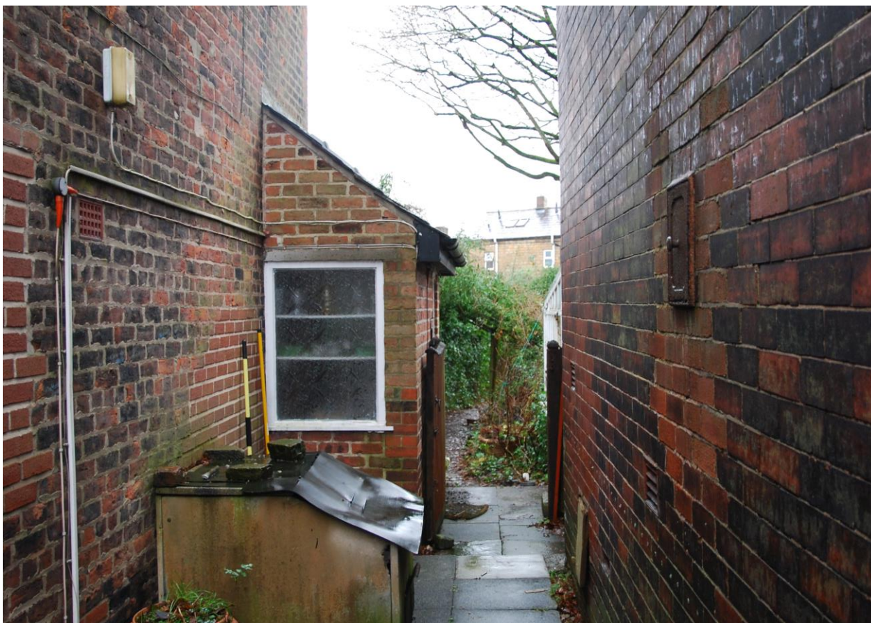
Fig 8. Rear of existing single storey rear extension showing obscure glazing.
