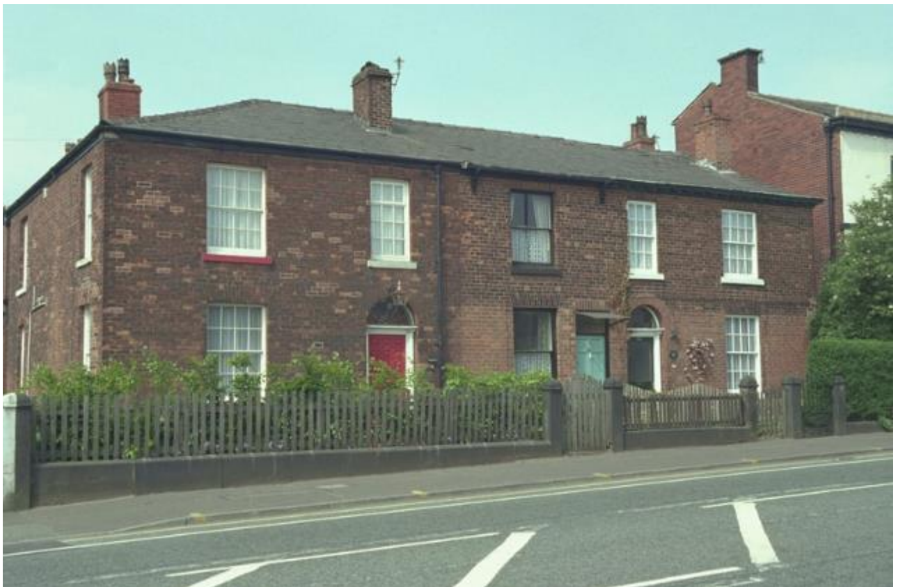
Fig 4. Image of 110, 108 and 108A Manchester Road taken from the archive of Historic England and the listing of the dwellings. Ref no IOE01/01663/30
