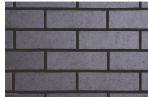
Brickwork - Staffordshire Blue Engineering Brick
