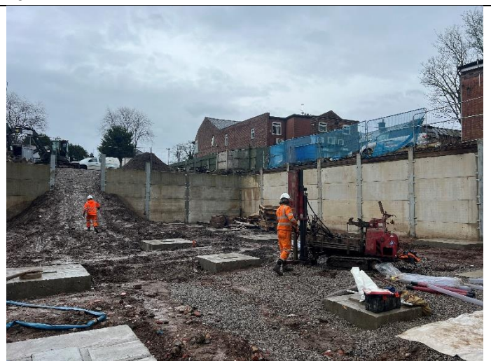
12: MW3 in progress
