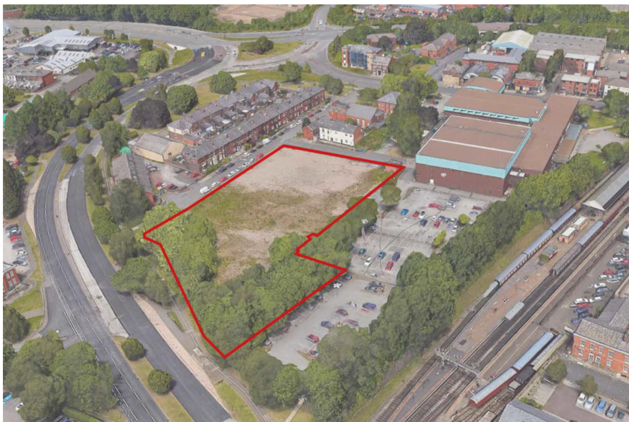
Existing Site Overview
