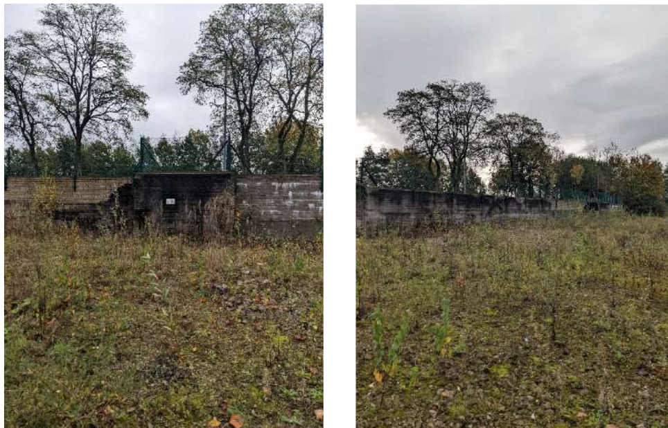
Figure 5: Photographs showing the retaining wall along the eastern site boundary.
