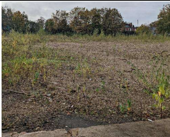
Figure 1 – The site with the concrete slab in the foreground, looking south.
