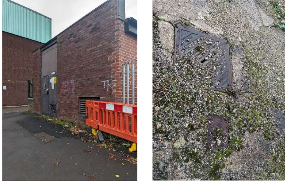
Figure 4: Photographs showing the off-site electricity sub-station near the north-eastern site corner (left) and manholes noted along the northern site boundary (right).
