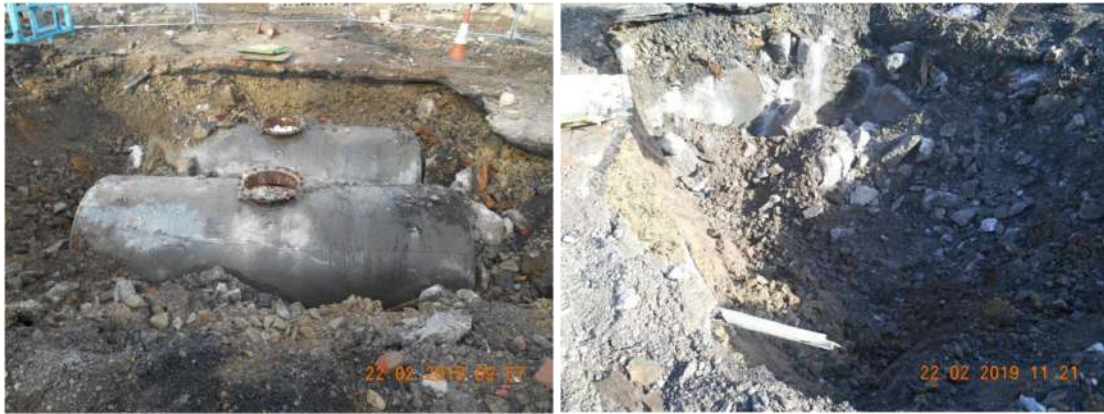
Figure 4 - E3P Photographs showing the tanks (left) and the exposed concrete cradle (right).
