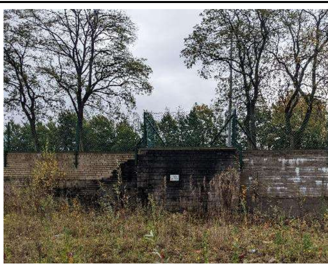
Figure 4 – The eastern retaining wall, looking east.
