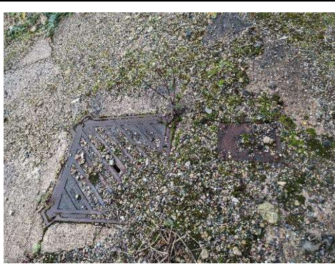
Figure 12 – Manholes along the northern site boundary, looking east.
