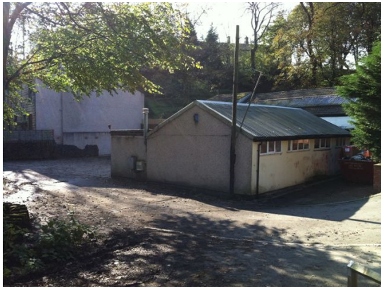
Photo 1 – Existing Site from NE
