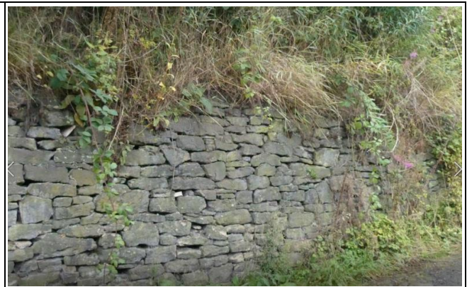
Retaining Dry Stone Walling to Eccles Street
