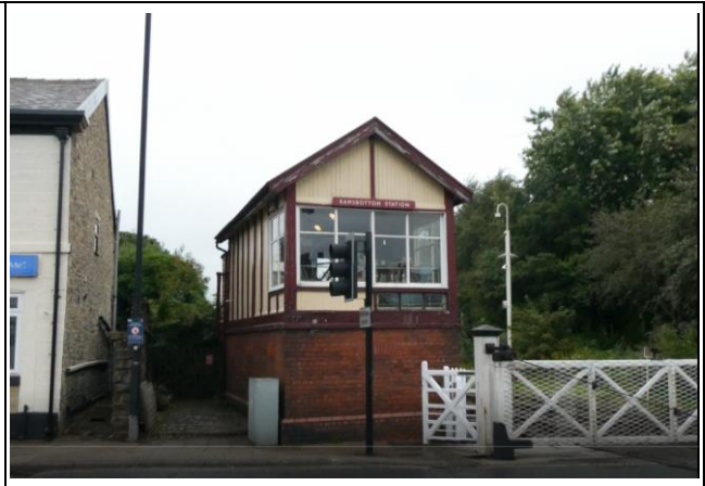
Railway Signal Box
