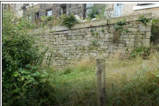
Dry Stone Walling to Houses on Douglas Street
