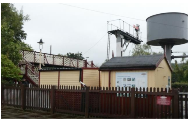
Cast Iron Footbridge Over the Railway
