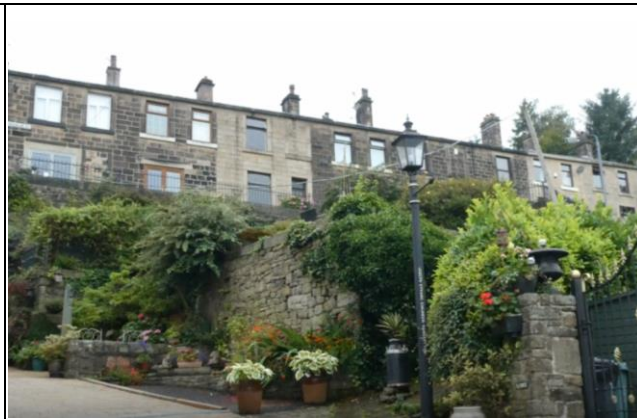
Milton Lane Leading to Houses at Douglas Street
