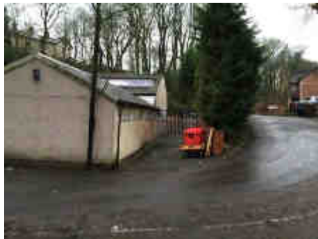
Photograph 6 (P6) View of existing works with elevated ground to the west visible.
