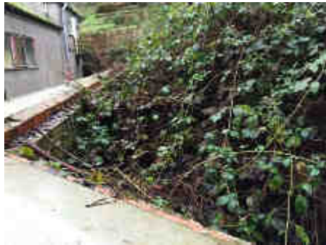
Photograph 4 (P4) Vegetated area present above the retaining wall to the west of the existing building.
