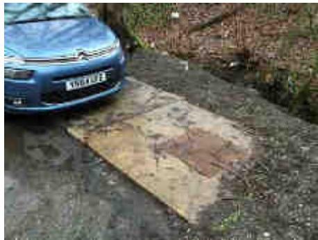
Photograph 8 (P8) Manhole covers associated with culverted watercourse visible adjacent to site.
