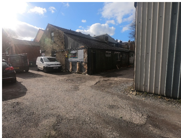
Existing stone building at the site entrance
