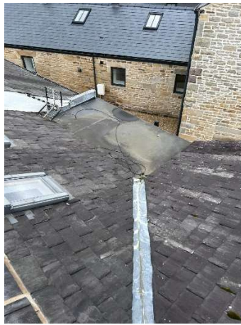
photos showing two existing flat roofs
