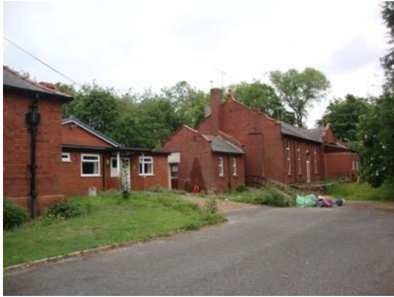
Fig 3 general view of buildings
