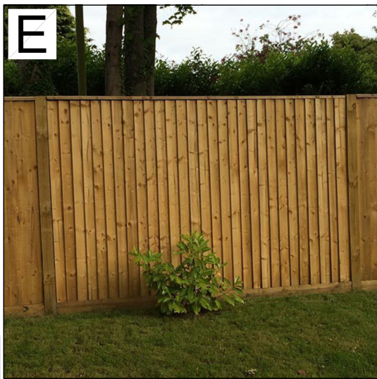
Image E: Closeboard timber fencing
