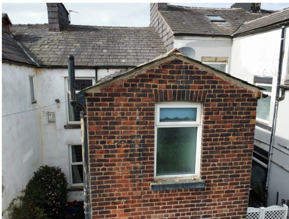
Photograph 2. Rear roof slope and proposed dormer will not create overlooking issues.
