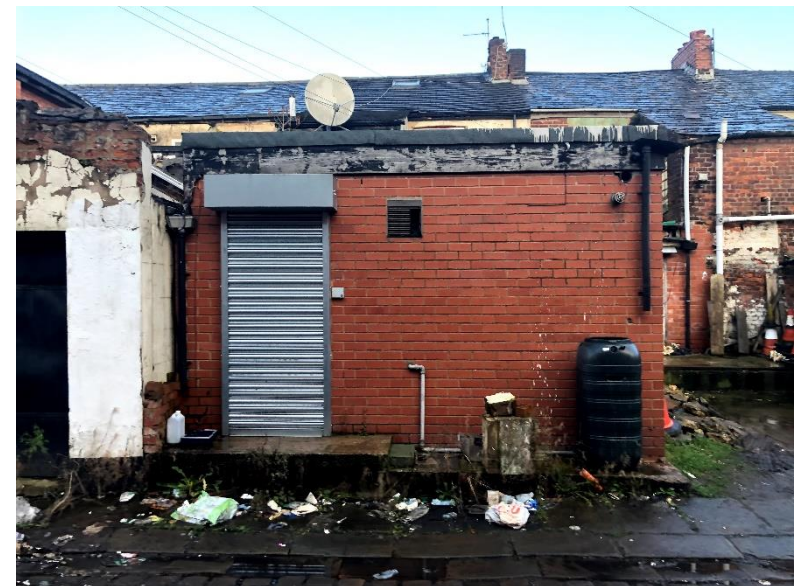
Figure 3: 88 Rochdale Road – Existing Rear Extension
