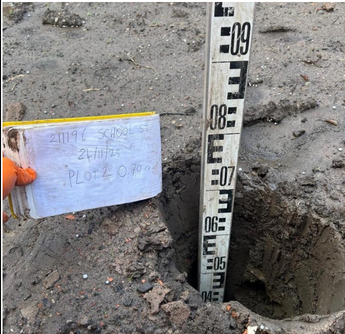
Plot 2: Overview of excavation
