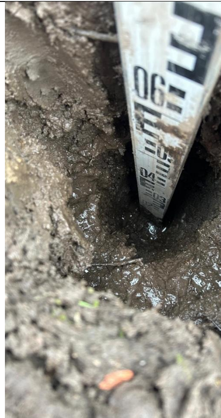
Plot 62: Internal View of excavation
