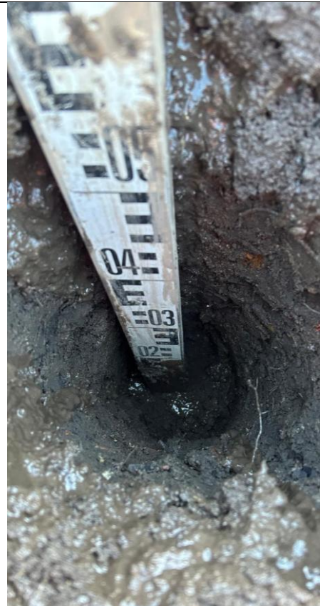
Plot 65: Internal View of excavation
