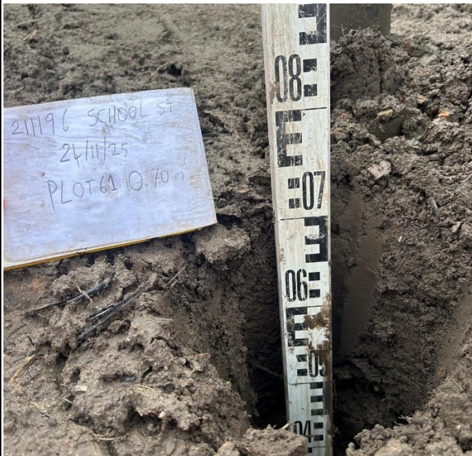
Plot 61: Overview of excavation
