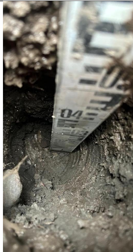
Plot 60: Internal View of excavation
