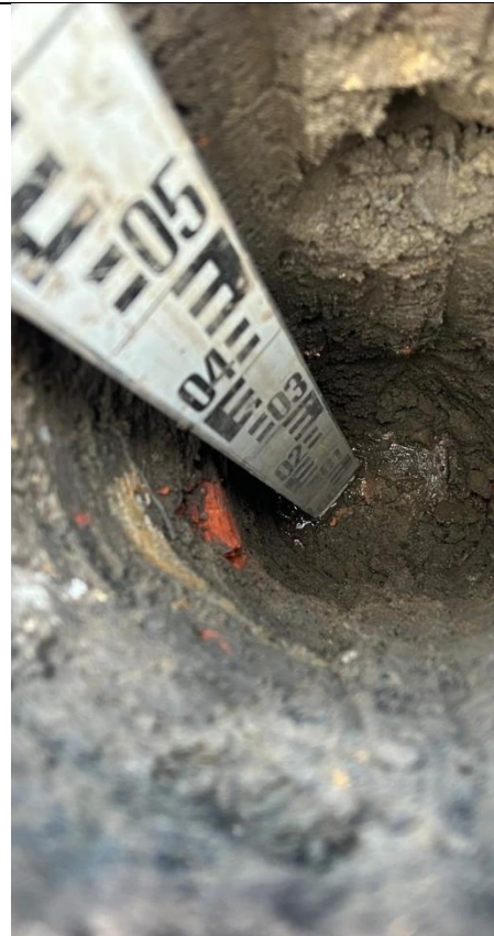
Plot 2: Internal View of excavation
