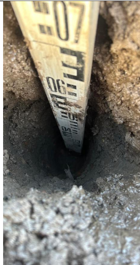
Plot 64: Internal View of excavation
