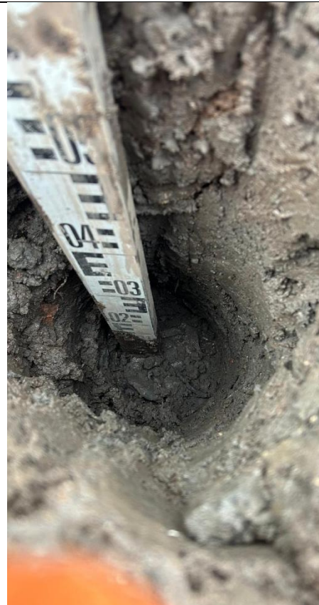
Plot 63: Internal View of excavation
