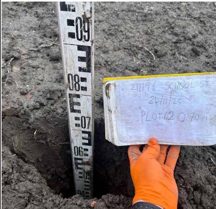
Plot 62: Overview of excavation
