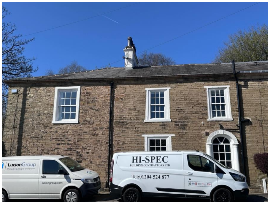
Fig .1, Barwood House
