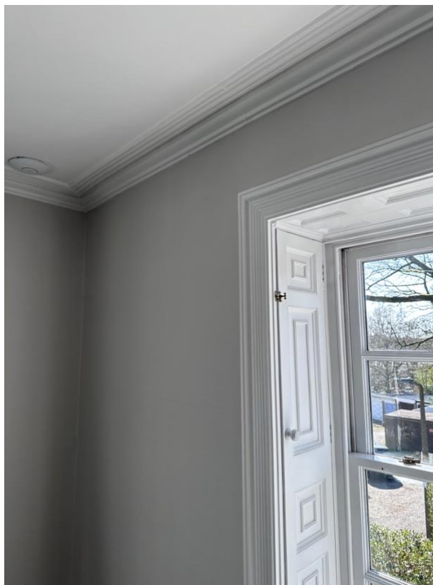
Fig 2, Image showing approx. location of the ensuite against existing window and coving to be scribed around and protected.
