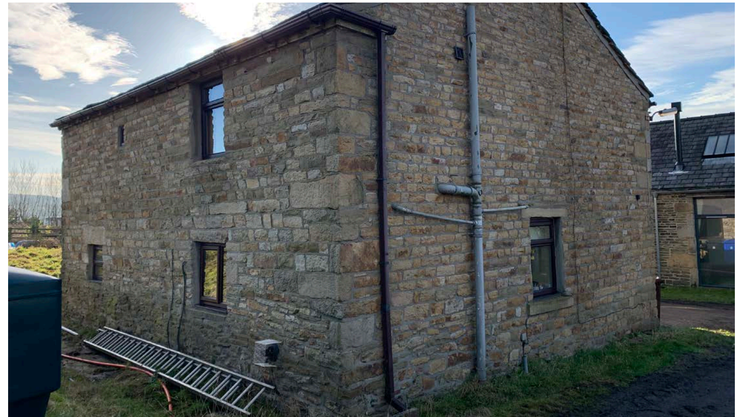
Above: Existing Property Rear (Faces Bury Old Road)
