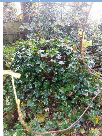
Photograph 6: Brick-Walled Hole (Possible Shelter Access)
