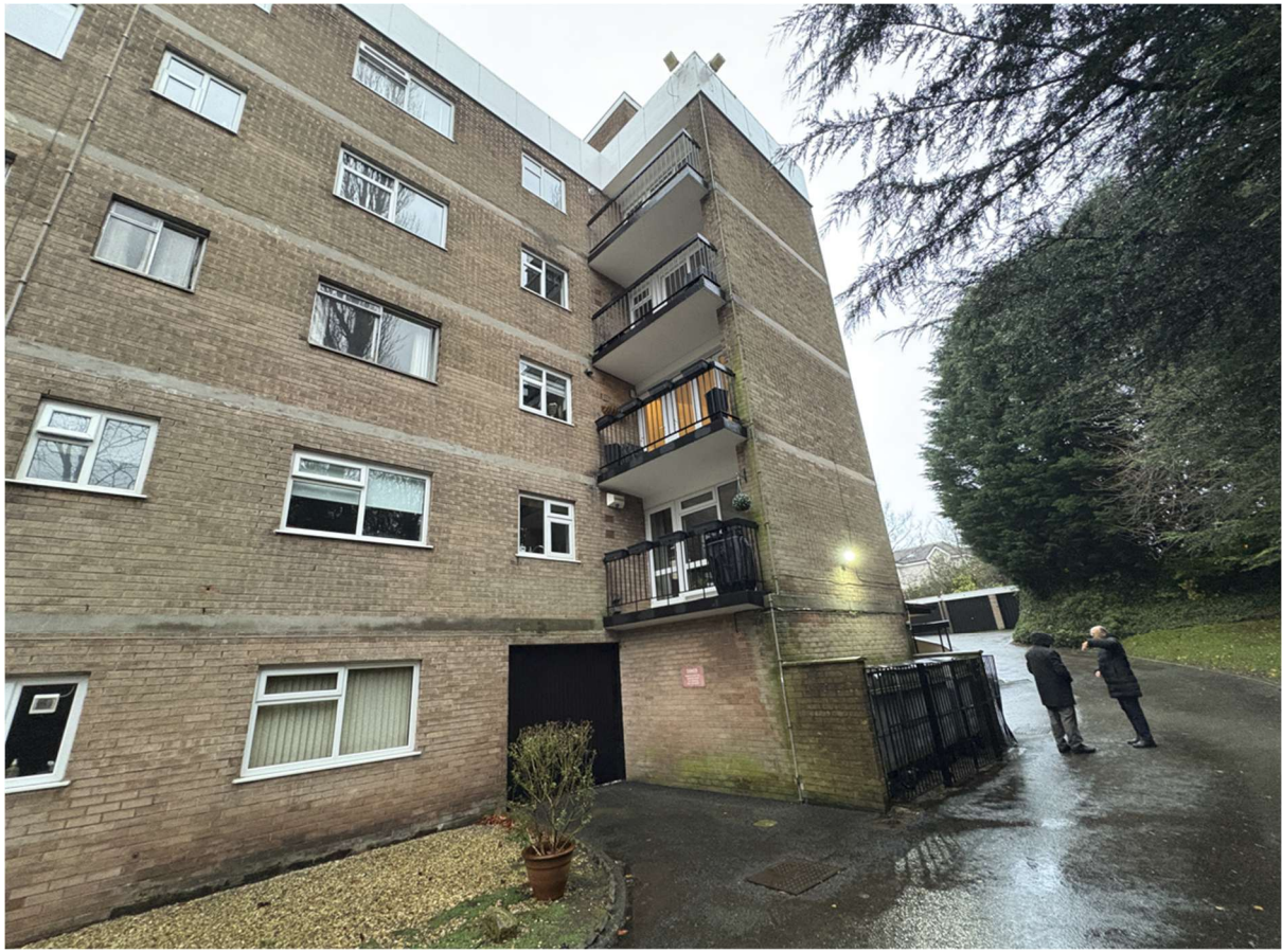
Photo of west elevation
