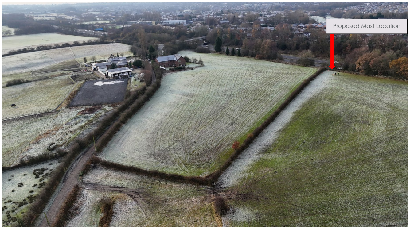
Figure 1: Proposed site location with the motorway in the background
